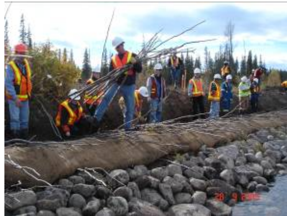
Vegetated mechanically stabilized earth (VMSE) Pembina River, 2005
