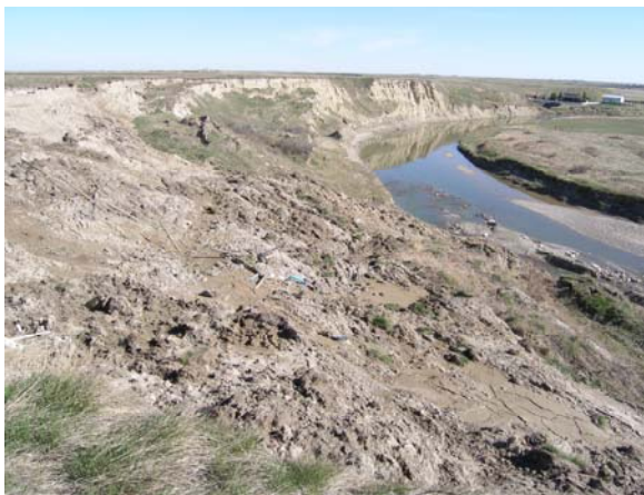
Willow Creek site, before - 2006
