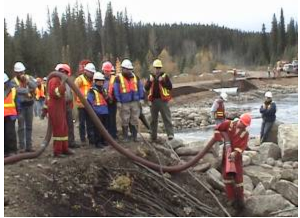
Placing blown-on compost blanket
