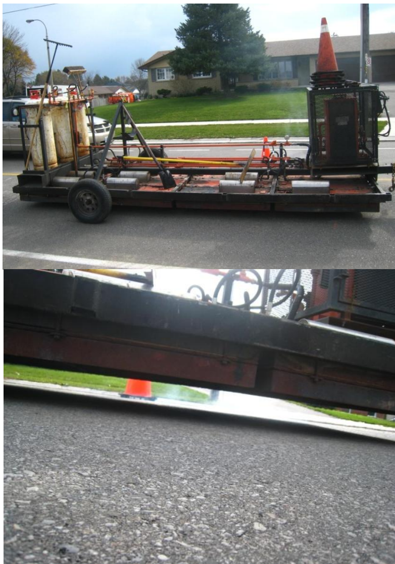
Figure 2 – Infrared Heater Softening a Cracked Area
