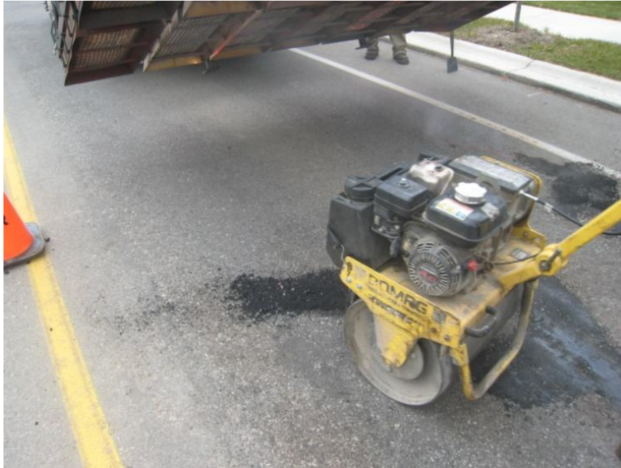
Figure 3 – Compaction of Repaired Crack
