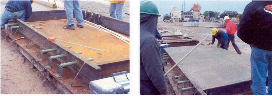
Figure 1. Precasting Michigan Method slabs, 3 dowel bars per wheel path
