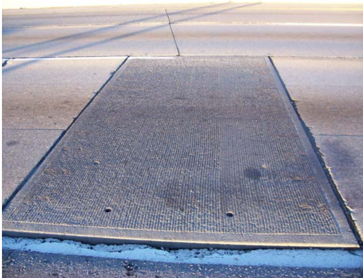
Figure 13 a) September 2007 and b) November 2009, Fort Miller Intermittent slabs performing well.
