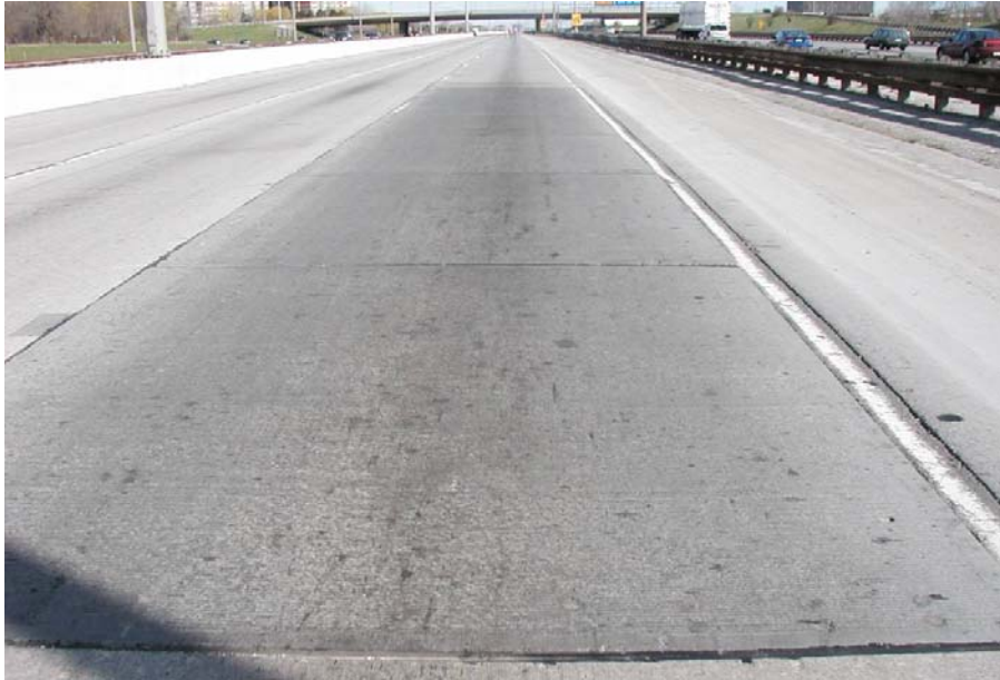
Figure 14. Performance of Fort Miller Continuous Slab repairs, May 2006.
