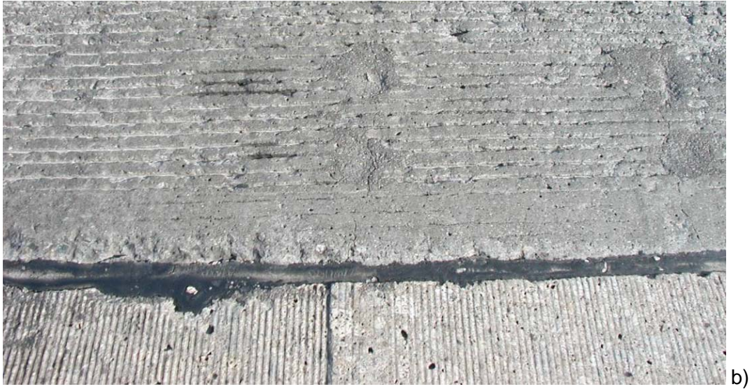
Figure 12 a & b) May 2006 observed slight cracking over dowel bars Fort Miller Intermittent slab.
