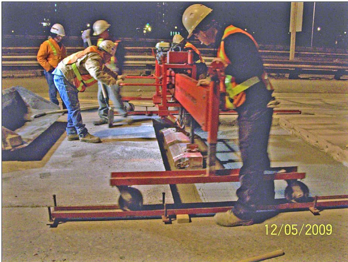
Figure 16. Precision grading equipment implemented on two contracts in 2009.
