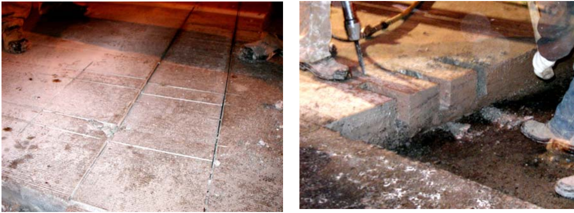
Figure 2 a) Sawcutting and b) Excavation of Dowel Bar Slots for Michigan Method
