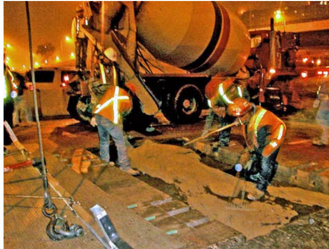
Figure 4. Use of flowable fill as a levelling material.
