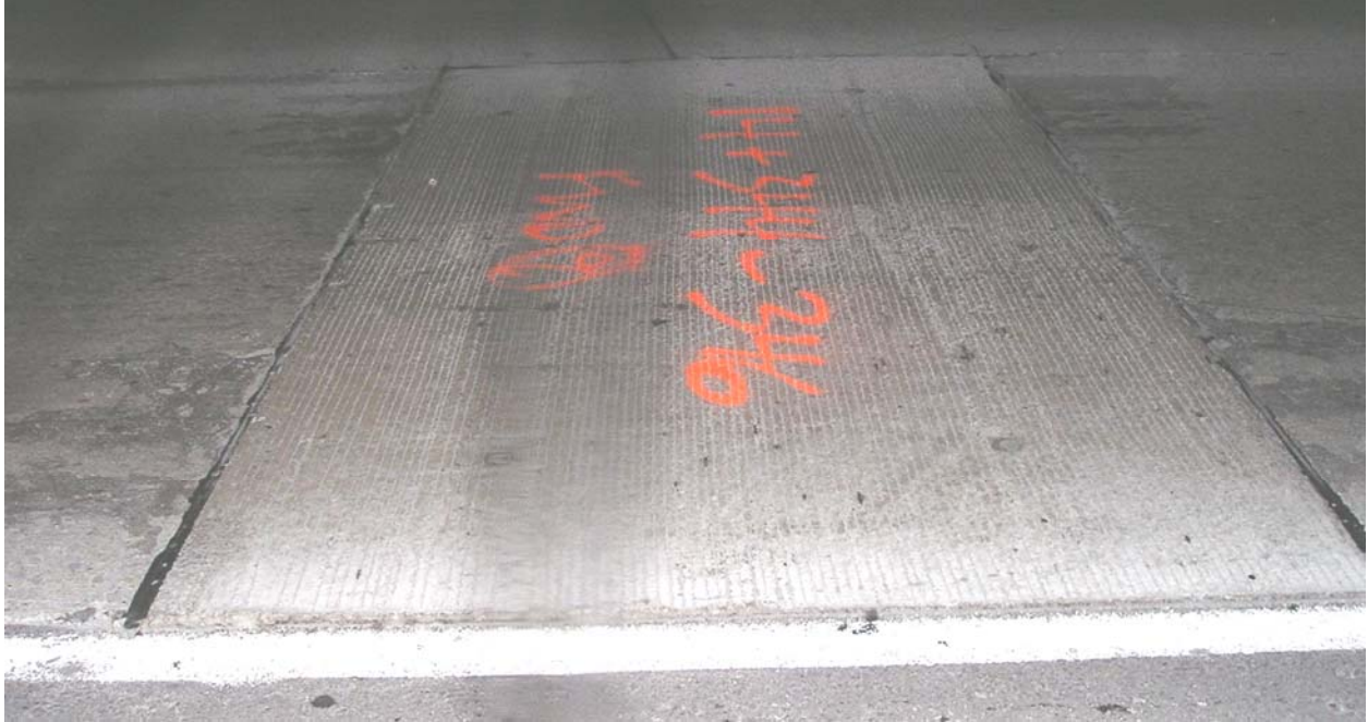
Figure 9. Michigan Method precast slab, June 2005.
