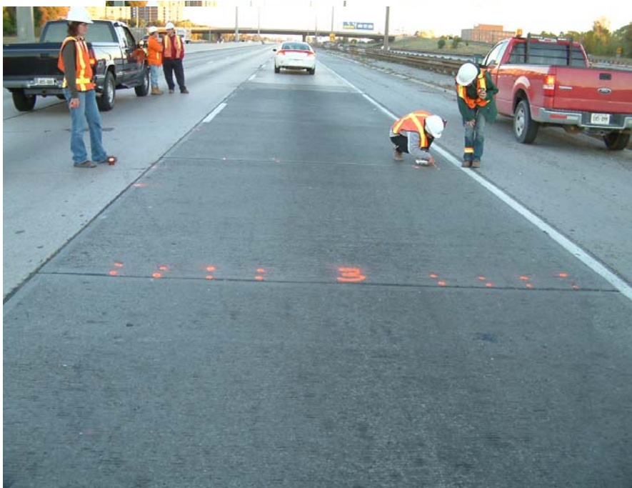
Figure 15. Performance of Fort Miller Continuous Slab repairs, September 2007.
