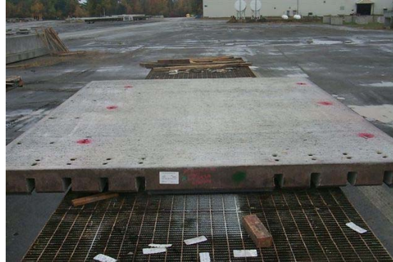
Figure 6. Four block-outs per wheel path are cast into the Fort Miller intermittent slabs.
