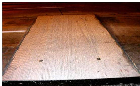
Figure 5. Completed Michigan Method slab repair
