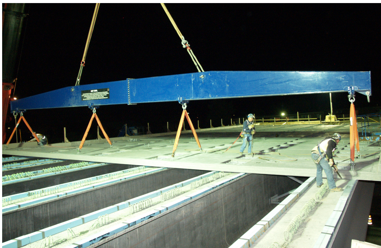
Glenmore Trail / 37 Street SW Interchange – Stage 1 Detour, Setting Precast Deck Panels, August 24 10:18 PM
