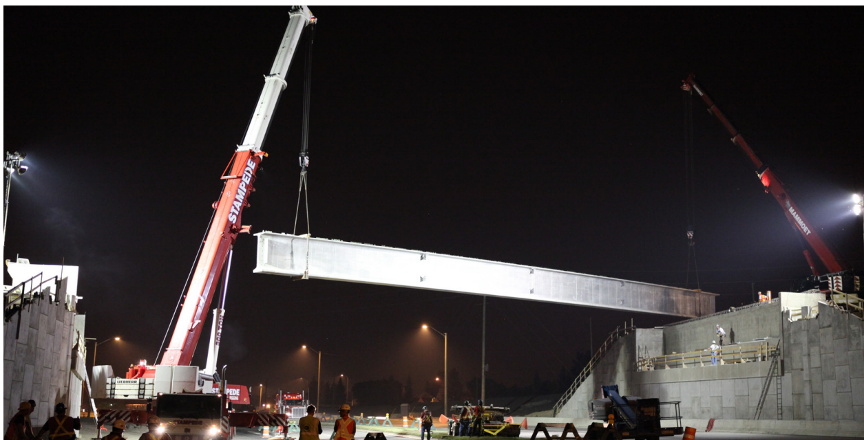
Glenmore Trail / 37 Street SW Interchange – Stage 1 Detour, Setting First Precast Girder, August 19 10:35 PM
