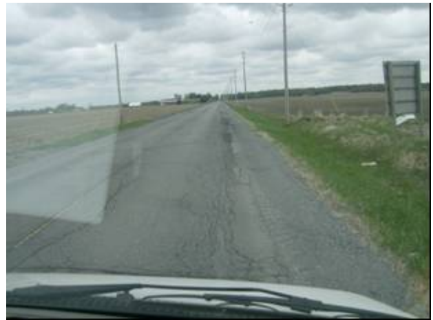
Figure 5: Alligator Cracking, Pre Construction (left) and Post Construction (right)
