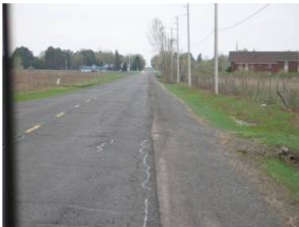
Figure 9: Transverse Cracking, Pre and Post Construction (left and right respectively)
