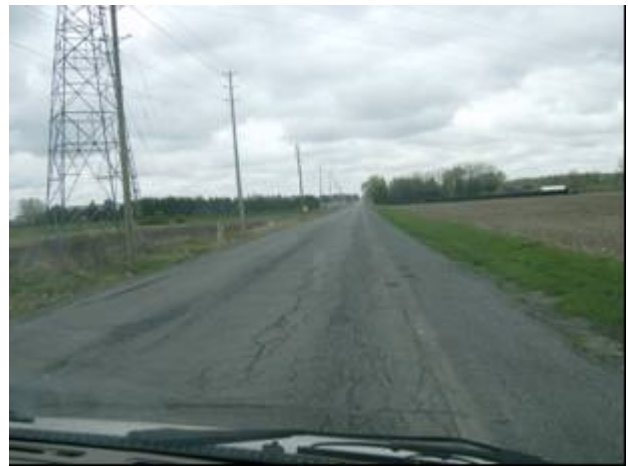
Figure 8: Alligator Cracking, Pre and Post Construction (left and right respectively)
