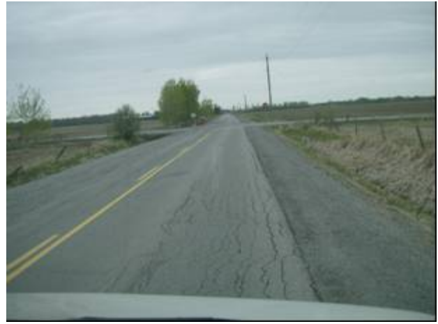
Figure 7: Edge Cracking, Pre and Post Construction (left and right respectively)
