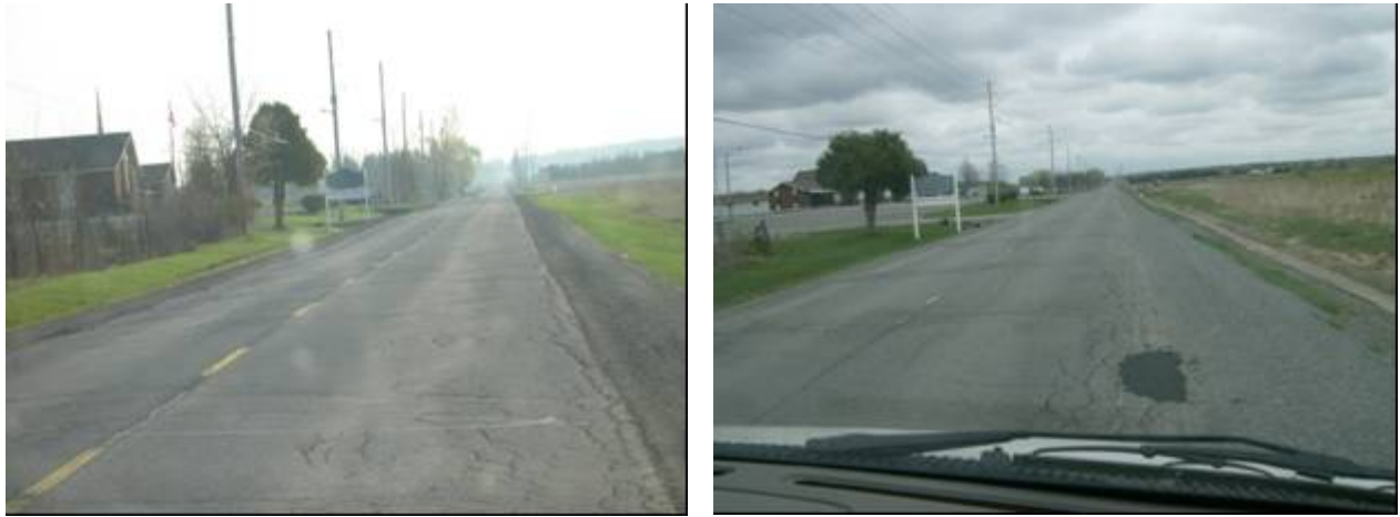
Figure 2: Alligator Cracking, Pre and Post Construction (left and right respectively)
