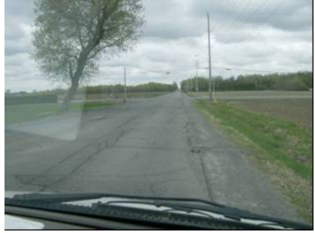
Figure 4: Transverse Cracking, Pre and Post Construction (left and right respectively)
