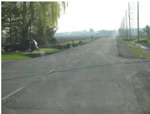
Figure 6: Transverse Cracking, Pre and Post Construction (left and right respectively)
