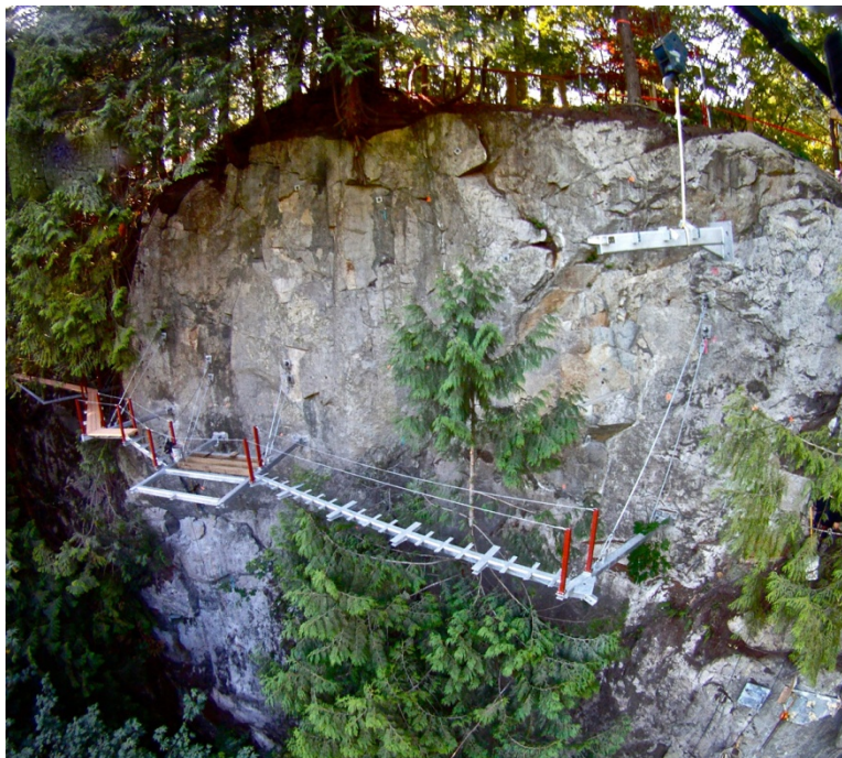
Figure 11 - Erecting the Steel Framework
