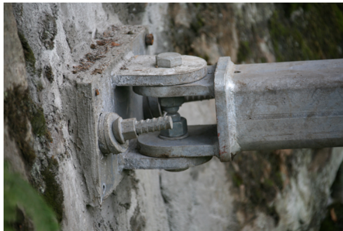
Figure 9 – Strut Beam Plate and Rock Anchors
