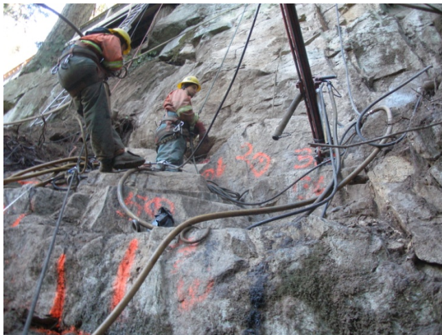
Figure 10 - Typical Rock Bolting Construction
