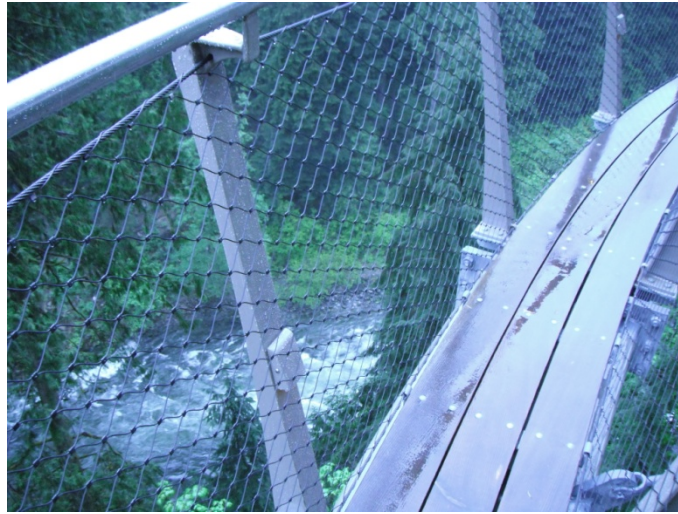
Figure 8 – Guardrail System
