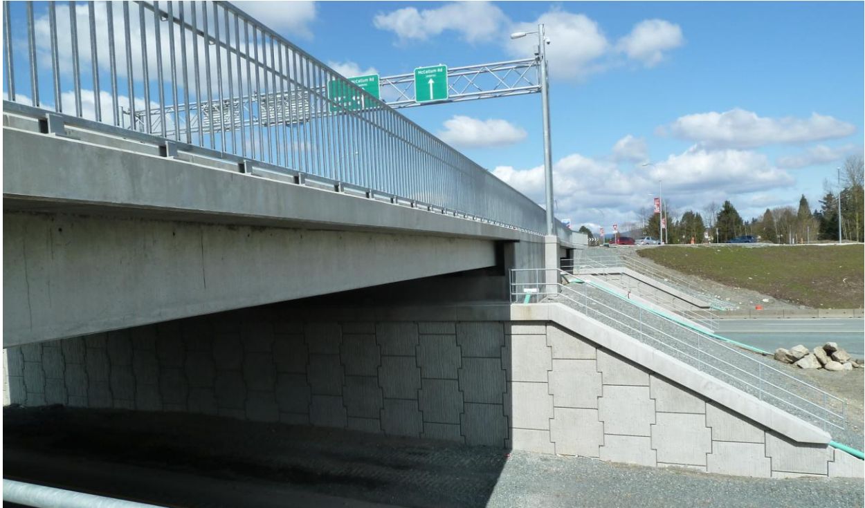
Figure 6: McCallum Underpass MSE Abutments
