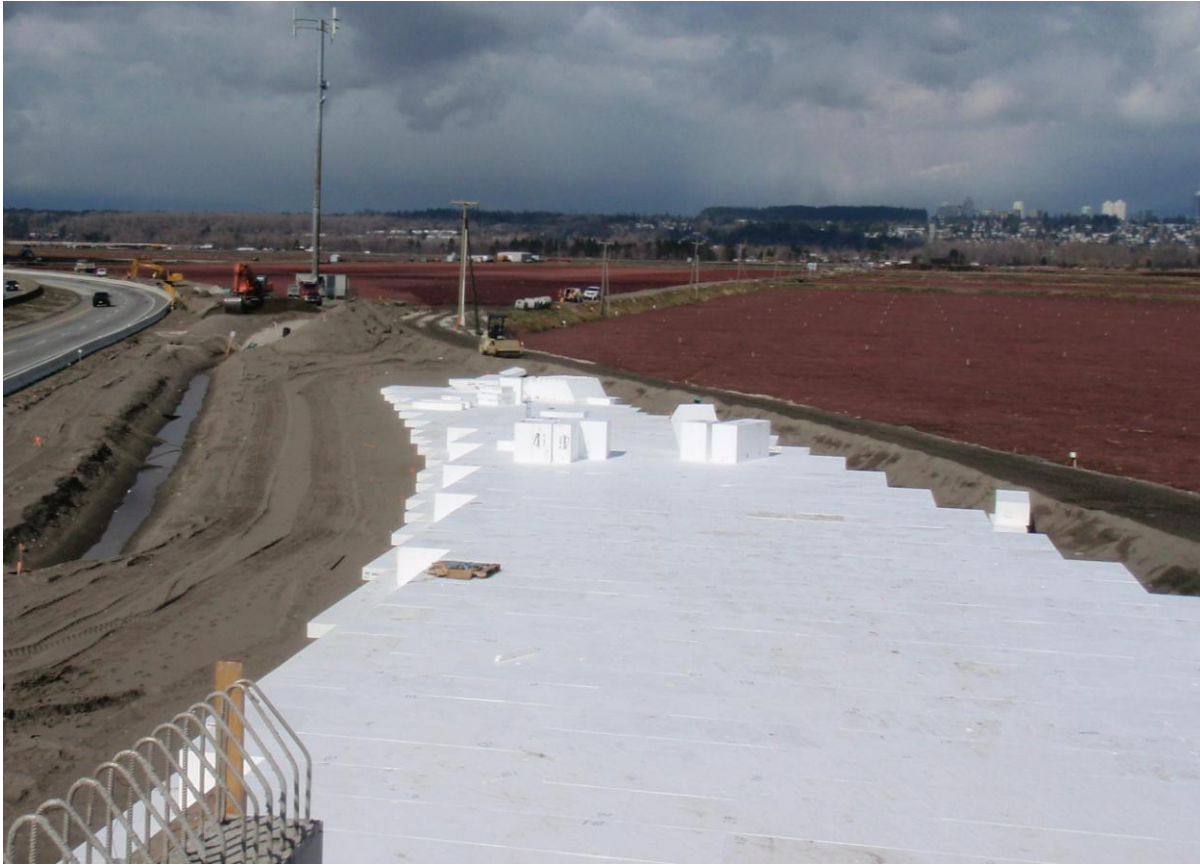
Figure 12: Nelson Flyover: EPS Fill Placement for North Approach Embankment
