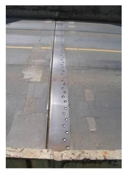
Figure 2: Deck deterioration over floor beams on each side of expansion joint.
