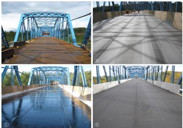
Figure 7: Deck construction sequence: A) panel bolting; B) grit blast surface; C) apply multi-coat waterproofing membrane; D) polymer-modified asphalt wearing surface.
