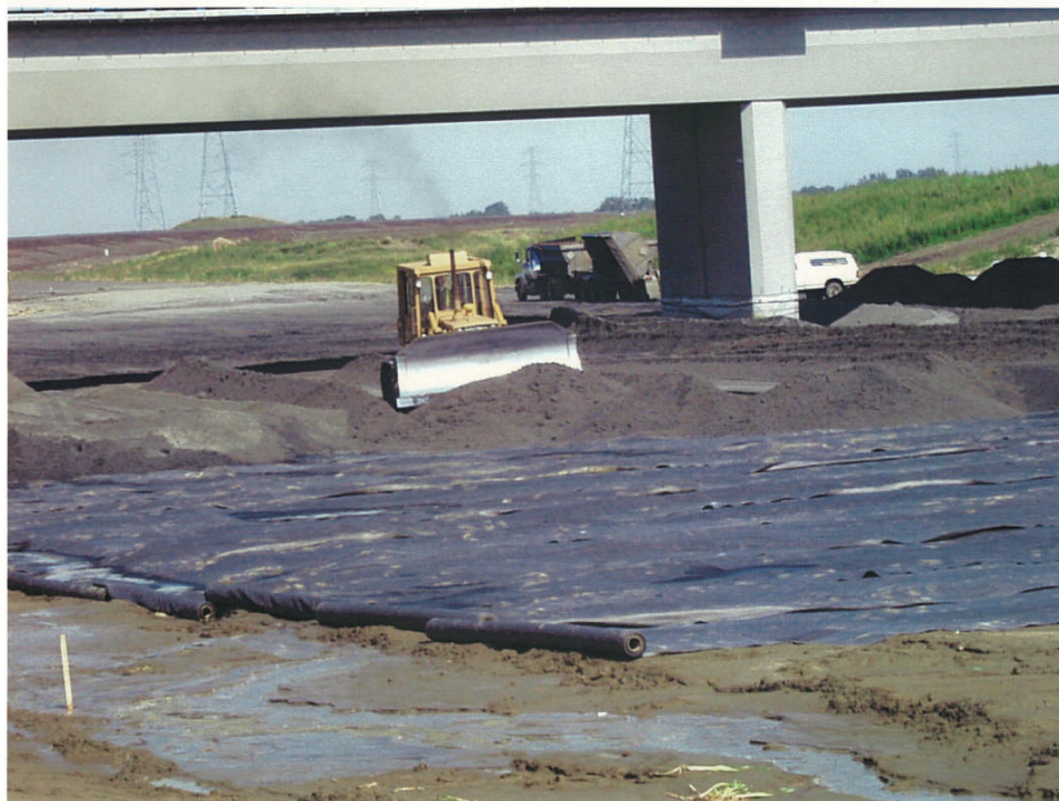
Photo 6: The Construction of a Bottom Ash Layer Directly on Weak Silt Subgrade
