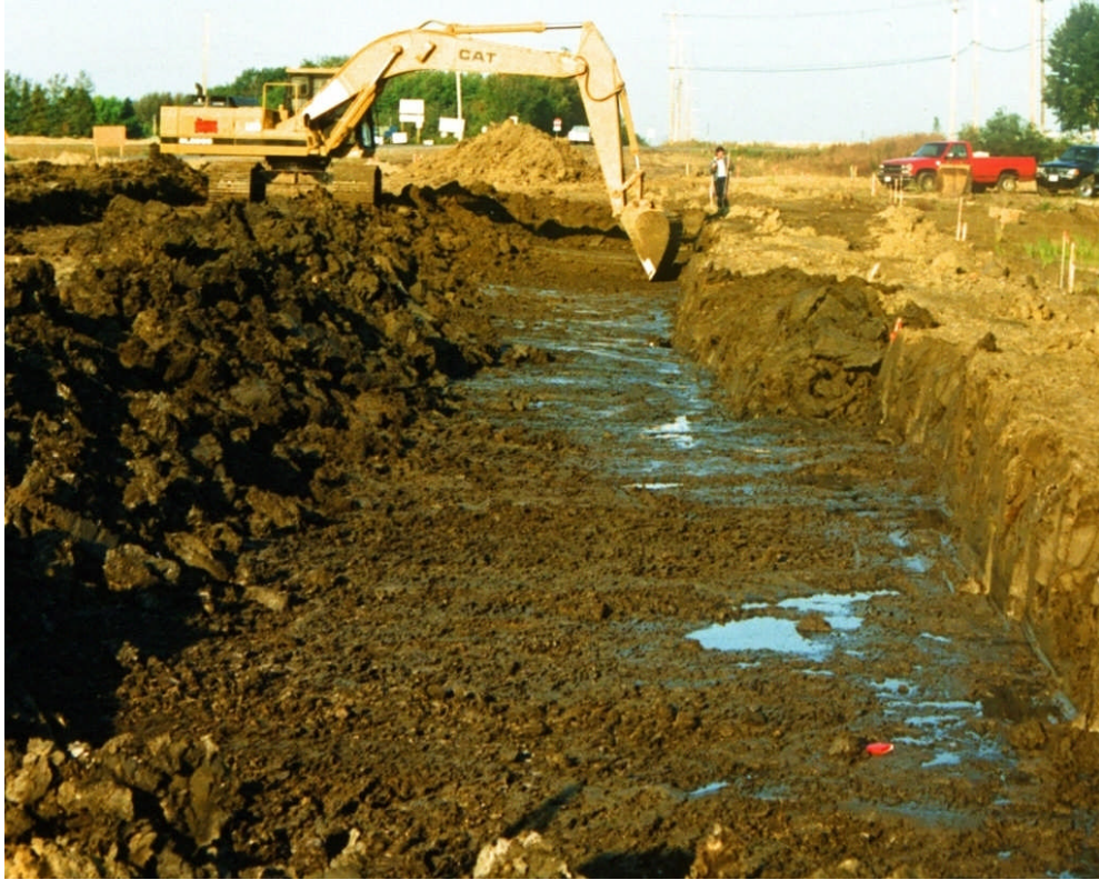
Photo 3: Exposing Weak Saturated Silt Layer
