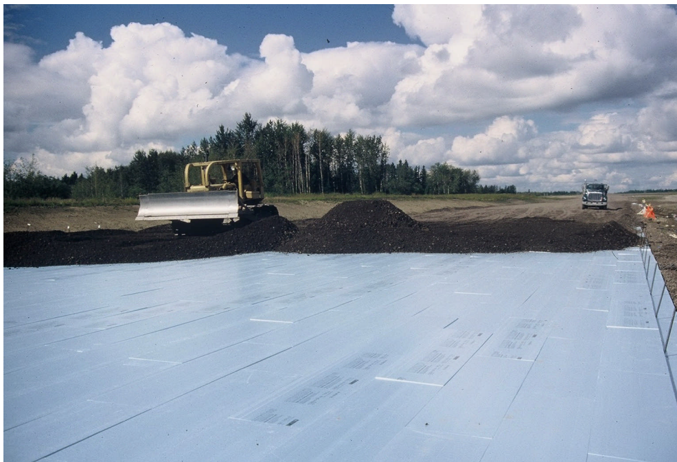
Photo 5: Base Course Being Placed on Polystyrene Insulation
