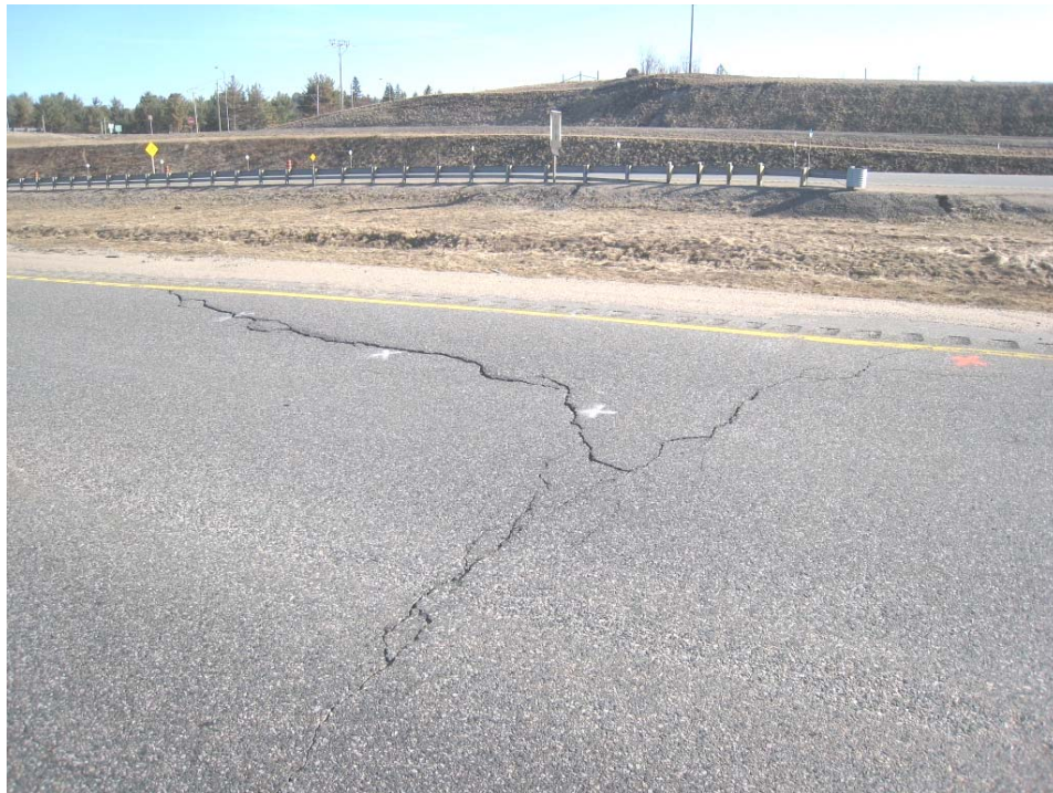
Figure 6. Frost Heave - Severe Meandering Crack
