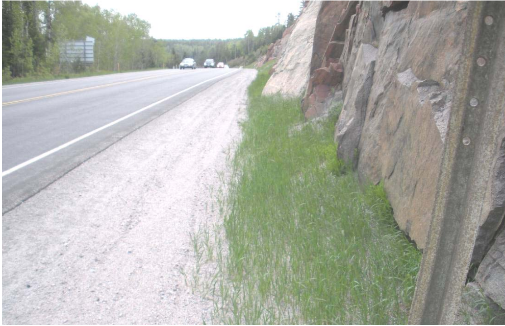
Figure 2. Poor pavement structure drainage in a rock cut area.
