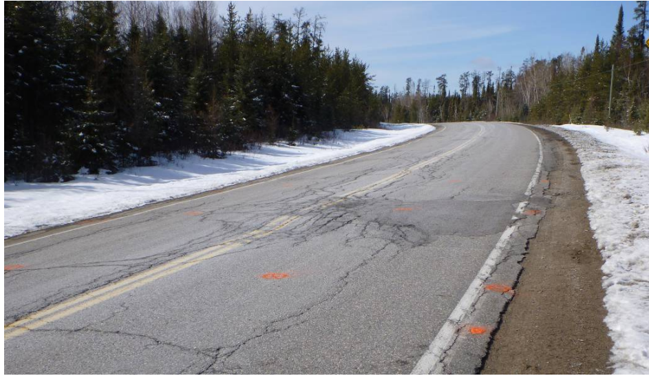
Figure 5. Transverse Frost Heave -Severe Distortion and Cracking
