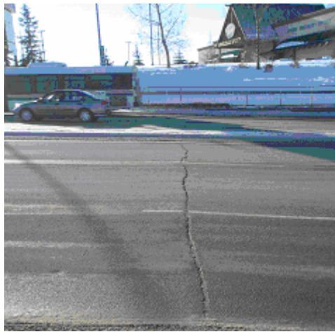
Figure 11. Crack due to Frost Heave
