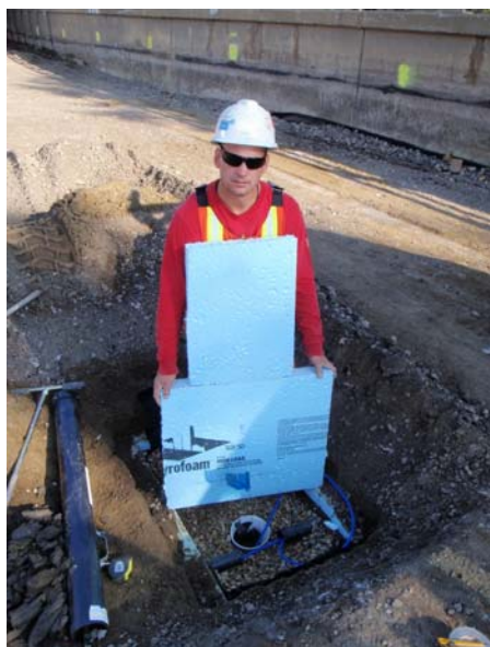
Figure 5. Thermistor Installation
