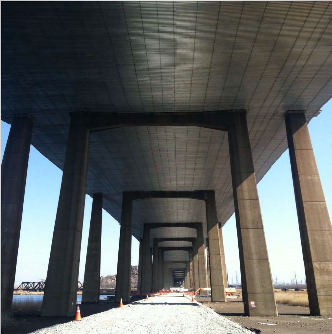
Hackensack River Bridge
