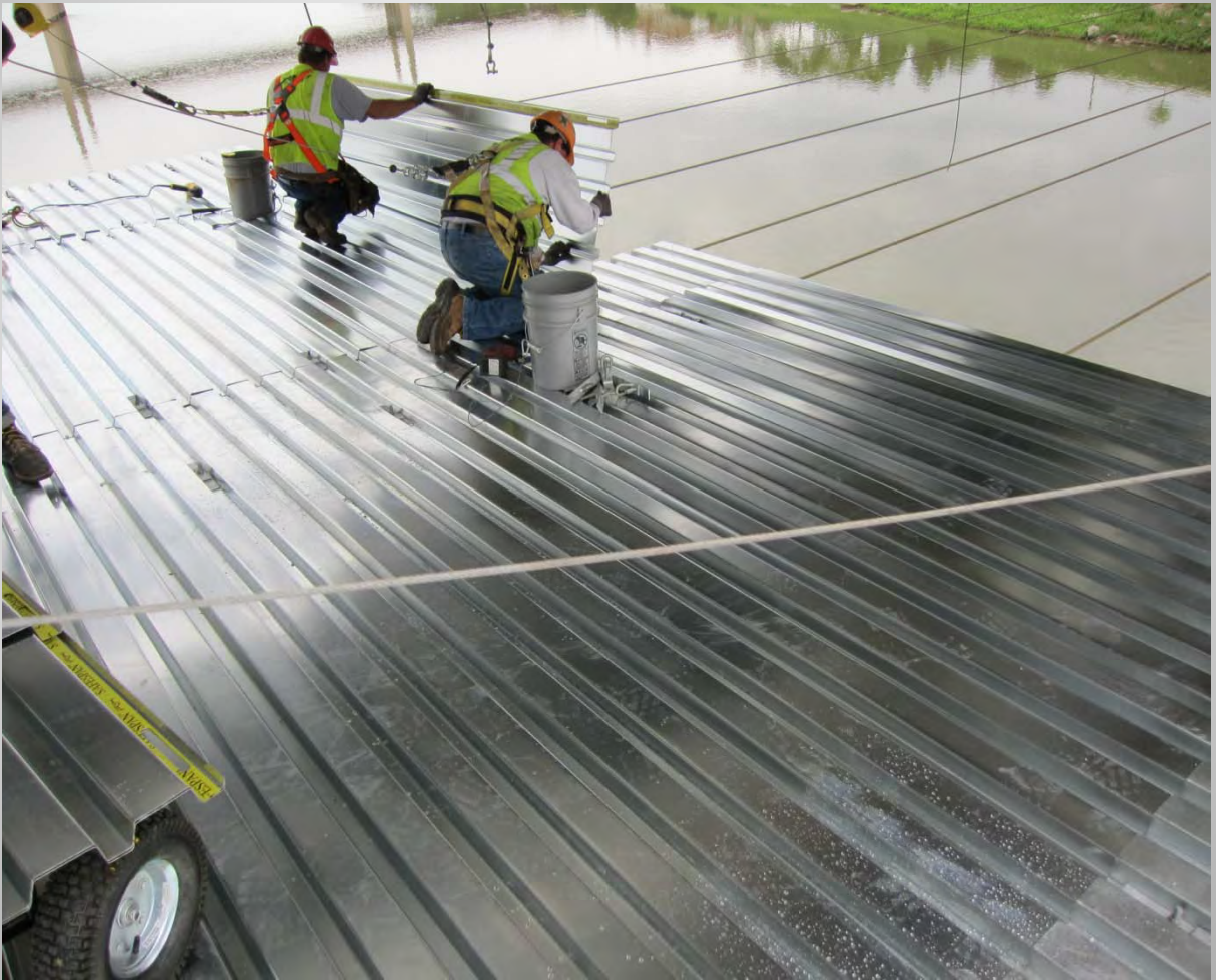
Laying Safespan Specialty Flooring Sections
