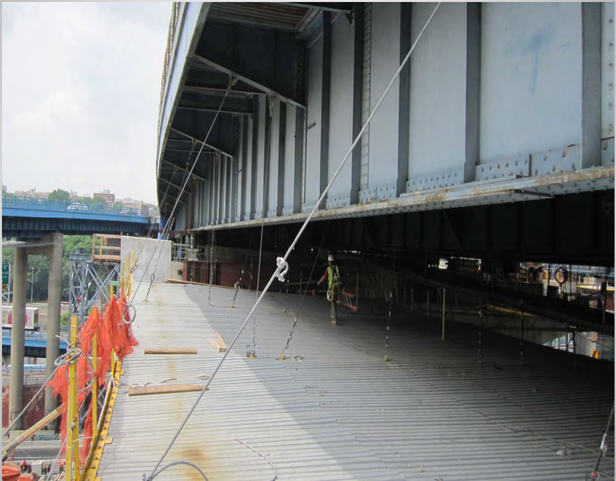
Alexander Hamilton Bridge
