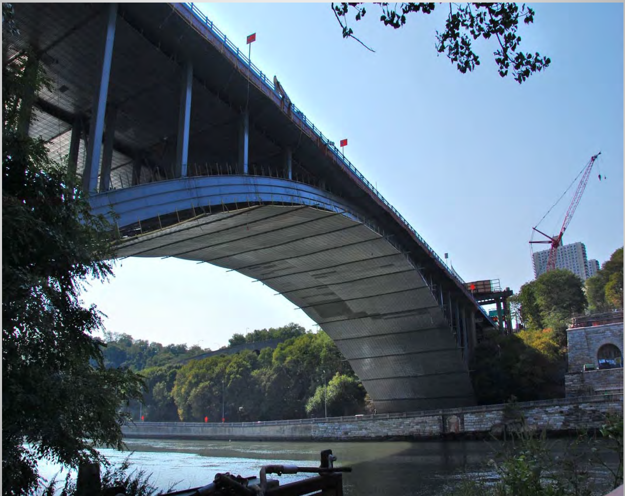
Alexander Hamilton Bridge
