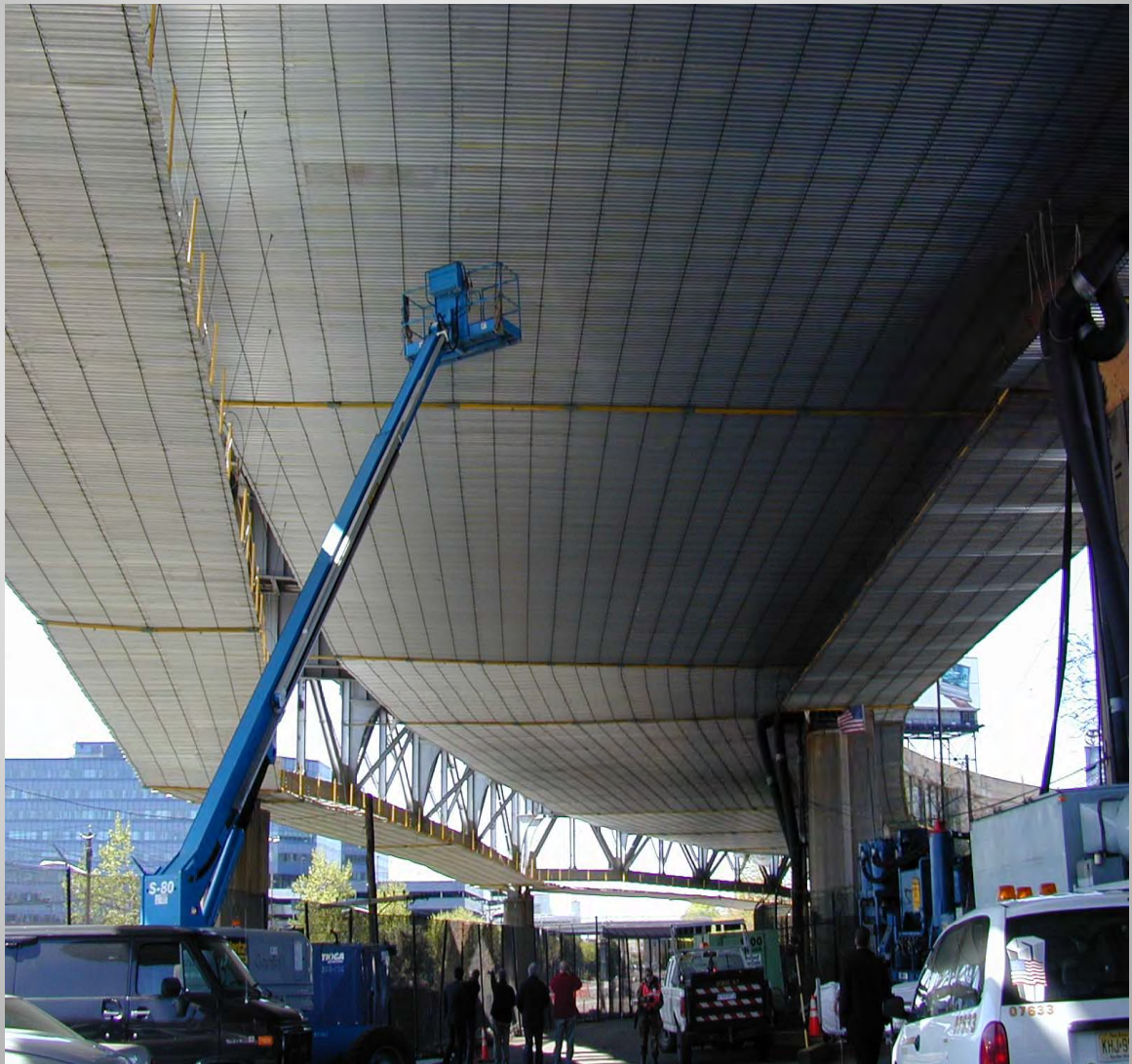
Lincoln Tunnel Helix
