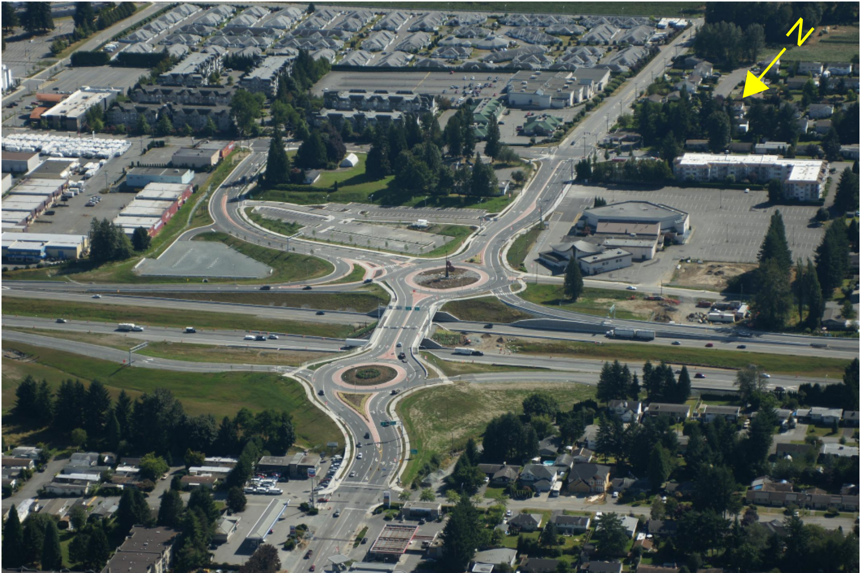
Looking South at the Completed Trans-Canada Highway and McCallum Road Interchange
