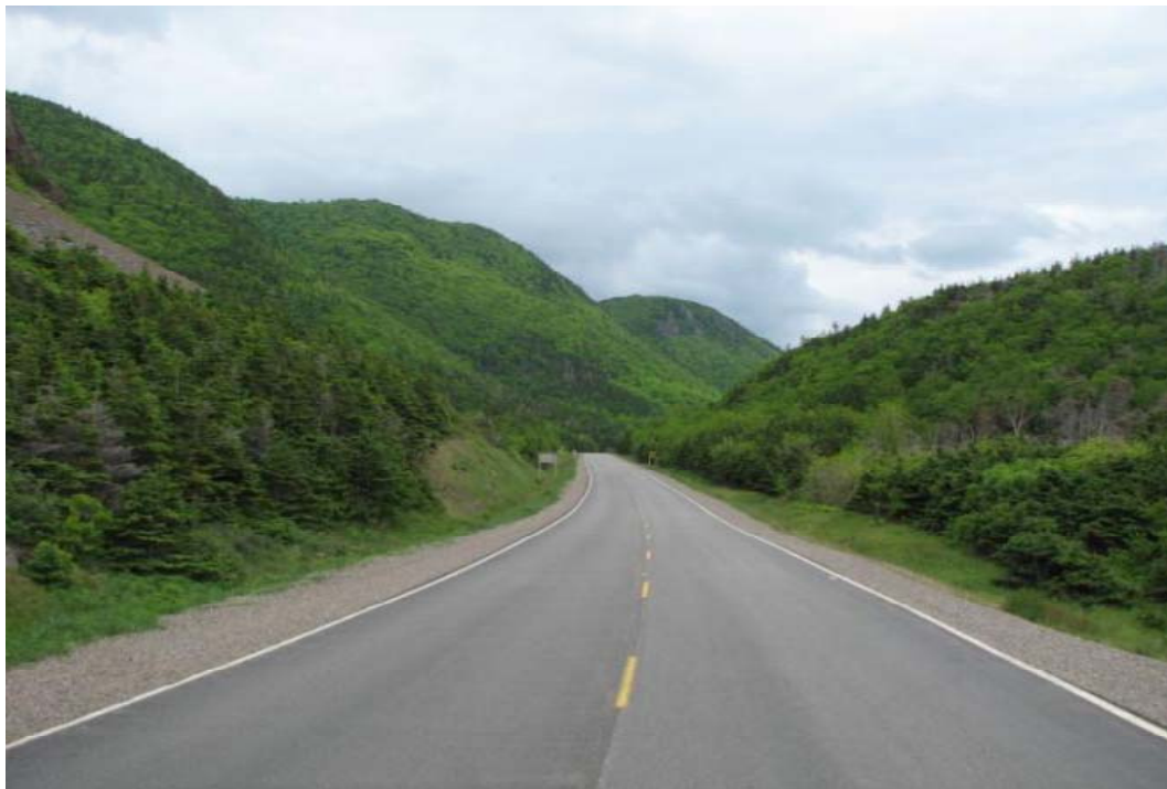
Figure 1 Pavement with a PCI 78
