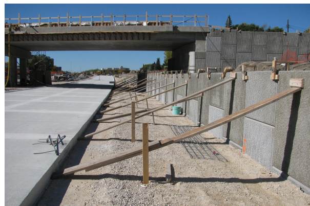
Photo 9: MSE Wall Construction Along CPT.
