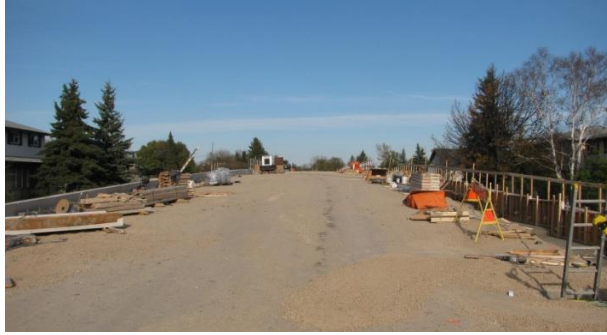
Photo 13: Rothesay Embankment Construction.
