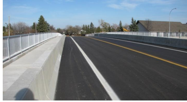
Photo 14: Rothesay Overpass and Roadway.
