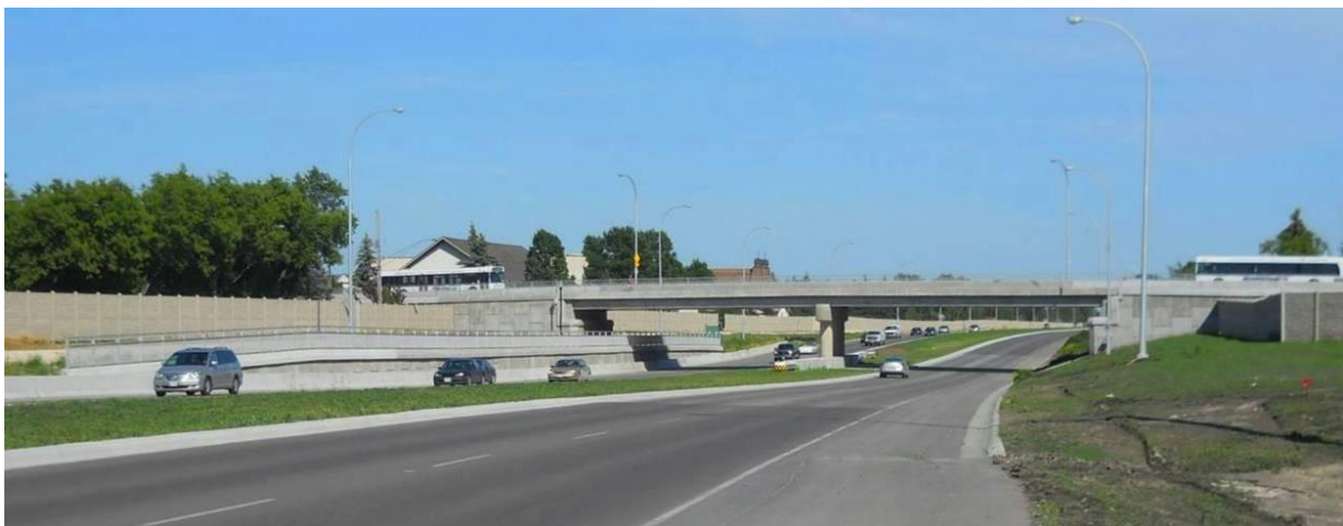
Photo 16: Rothesay St. Overpass and CPT Extension June, 2012.
