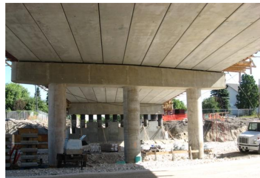
Photo 5: Underside of Overpass.
