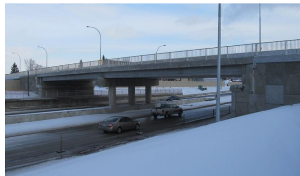
Photo 2: Rothesay St. Overpass and CPT, Dec. 2011.
