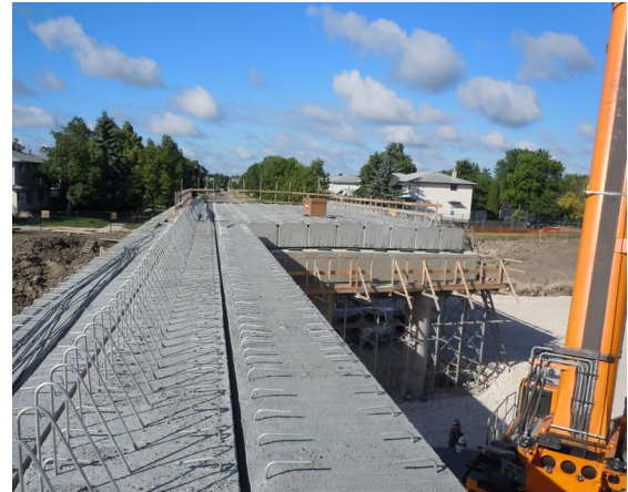
Photo 3: Erection of Precast Concrete Box Girders.
