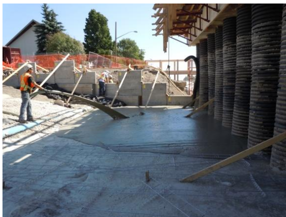
Photo 6: Pouring Cellular Concrete Behind Abutment Piles.
