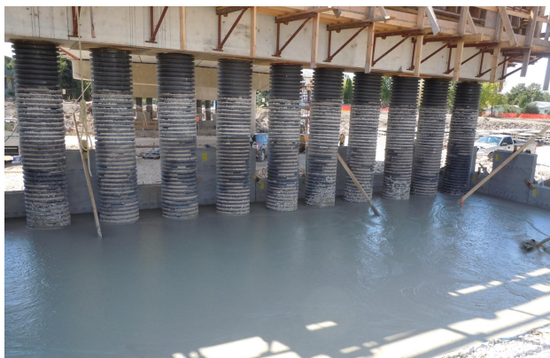
Photo 10: Liquid Cellular Concrete around Abutment Piles in HDPE Sleeves.
