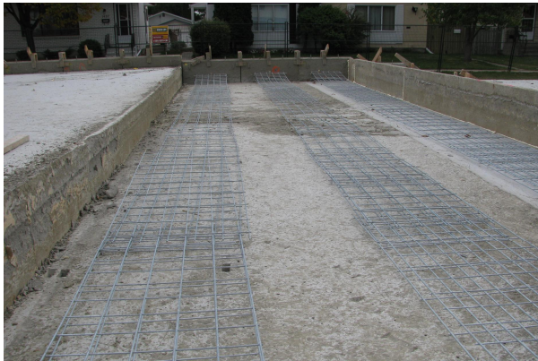
Photo 8: Galvanized Tie-Back Mats on Hardened Cellular Concrete.
