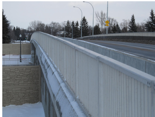
Photo 12: Aluminum Handrail and Noise Walls.
