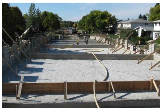
Photo 7: Stepped Cellular Concrete Embankment on Rothesay.
