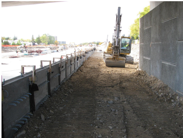
Photo 11: Multi-Use Pathway under Construction.
