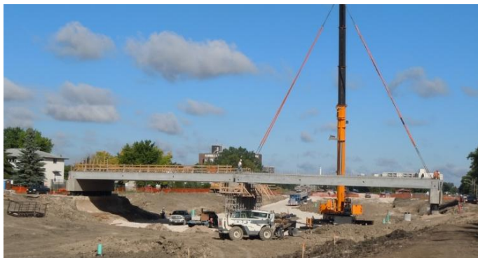
Photo 4: Erection of Precast Concrete Box Girders.
