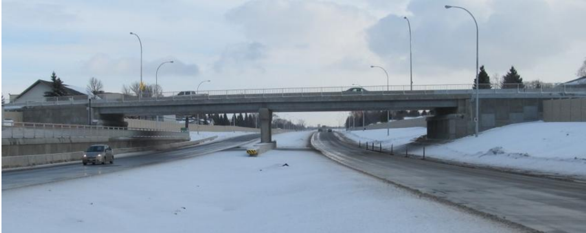
Photo 15: Rothesay St. Overpass and CPT Extension Open to Traffic.
