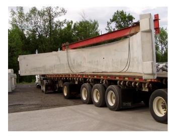
Figure 4. Moving Arch to Storage Yard
