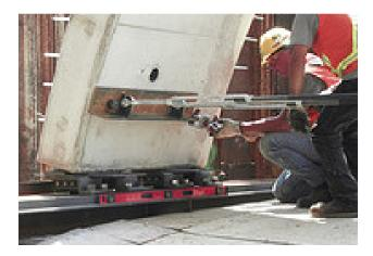
Figure 7. Landing on the Rollers
