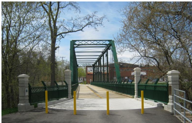
Figure 7 – View After Rehabilitation
