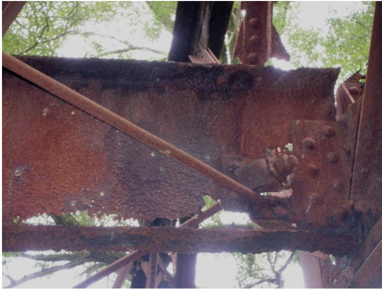
Figure 19 – Pony Truss Floor Beam Connection
