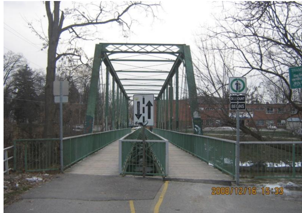
Figure 6 – View Before Rehabilitation
