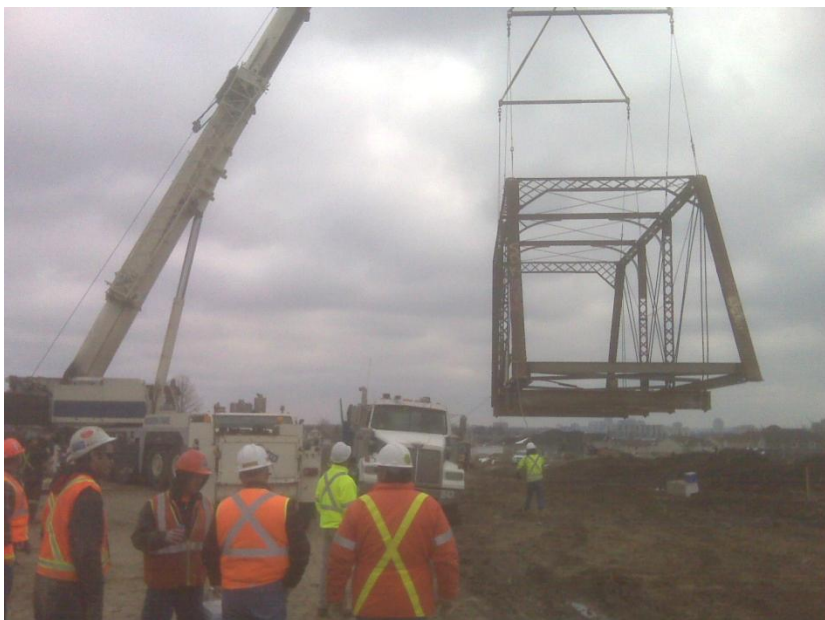
Figure 25 -- Truss Bridge Crane Lift
