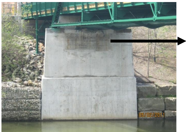
Figure 8 – Abutment Restoration
