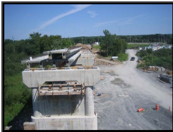
Figure 14: East Approach Deck Panel
