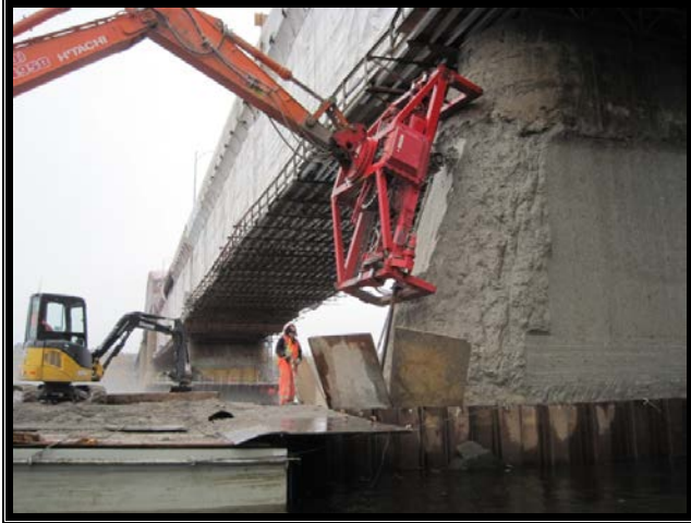
Figure 19: Concrete removal
