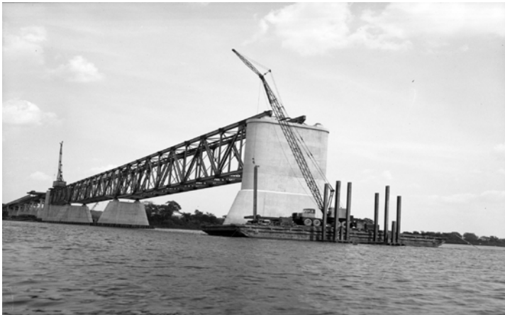
Figure 1: Bridge under construction circa 1958.
