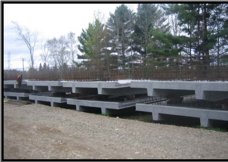
Figure 18: Precast panels stockpiled in storage yard
