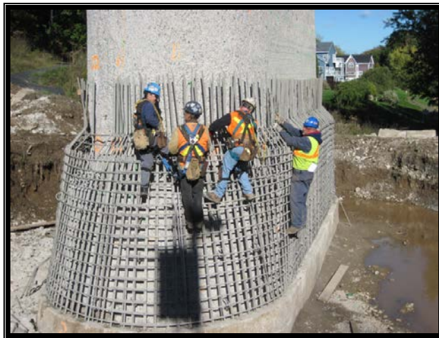
Figure 20: Installation of stainless steel reinforcement
