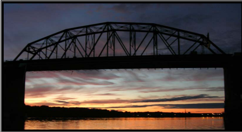
Figure 11: Through truss
