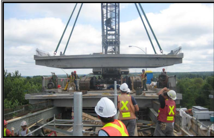
Figure 7: Installation of typical precast panel
