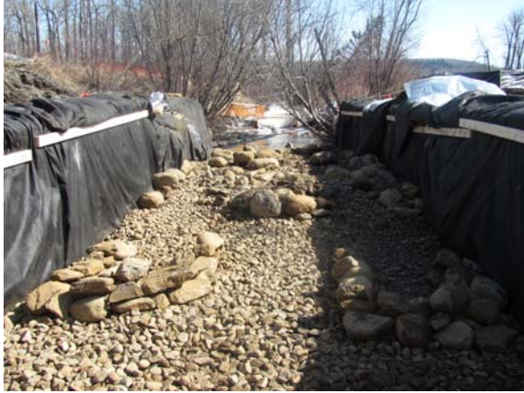
Temporary Streambed with J-Hook Vanes
