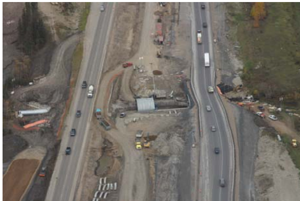
Construction under Core Lanes
