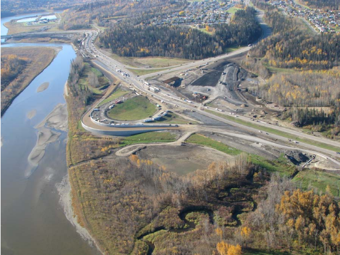
Figure 2: Conn Creek 500m North of Thickwood Interchange
