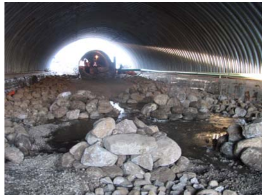
Permanent Streambed under Construction
