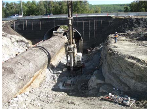
Neat and Dry Bed for Foundation Construction
