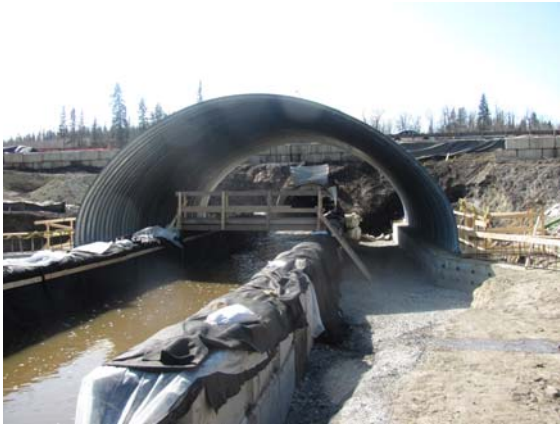
Assembled Culvert Extension
