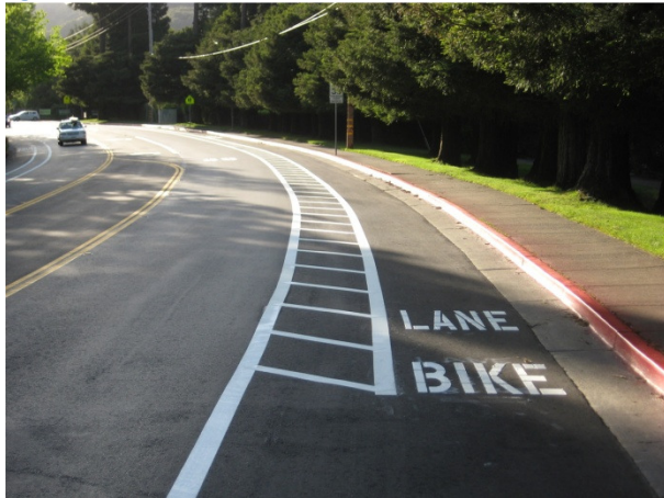
Figure 4 Buffered bike lane – Sir Francis Drake Boulevard, Fairfax, California
