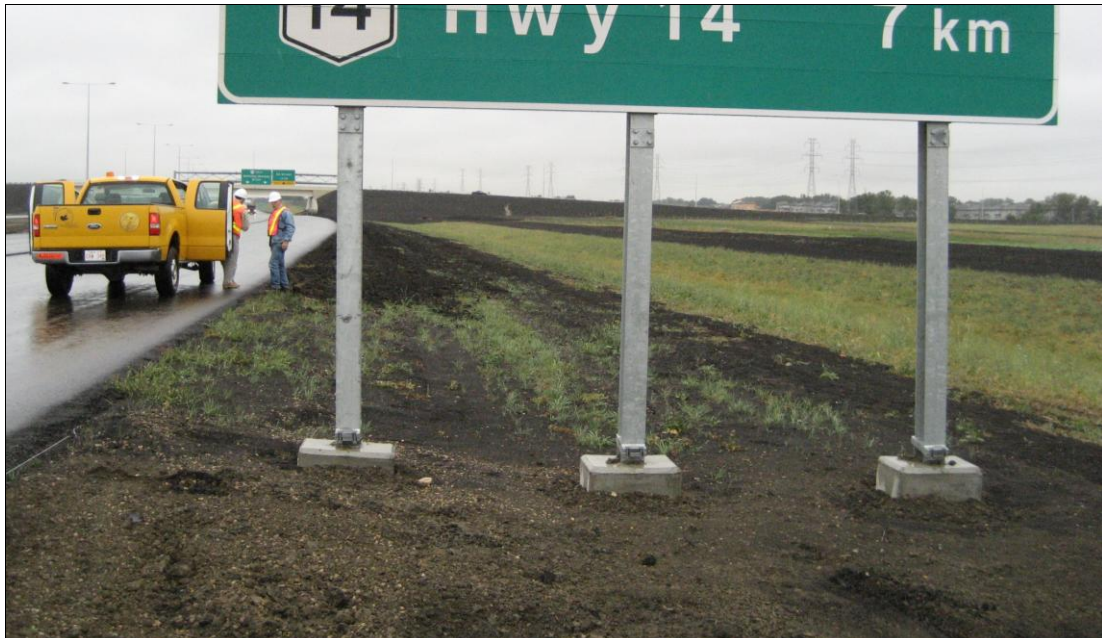
Figure 10: Over exposure of concrete footings
