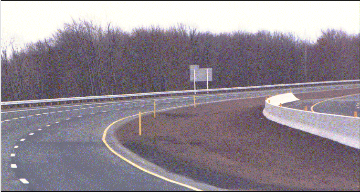
Figure 8: Delineation treatment along shoulder and on concrete barrier
