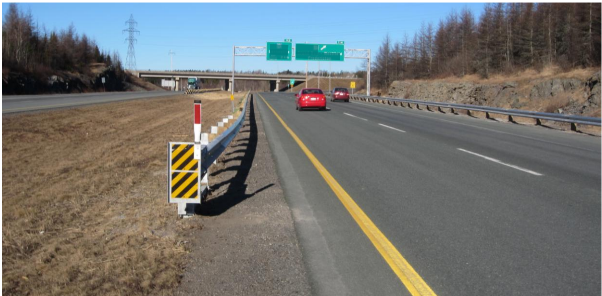
Figure 7: Improper orientation of Object Marker on a guiderail end terminal
