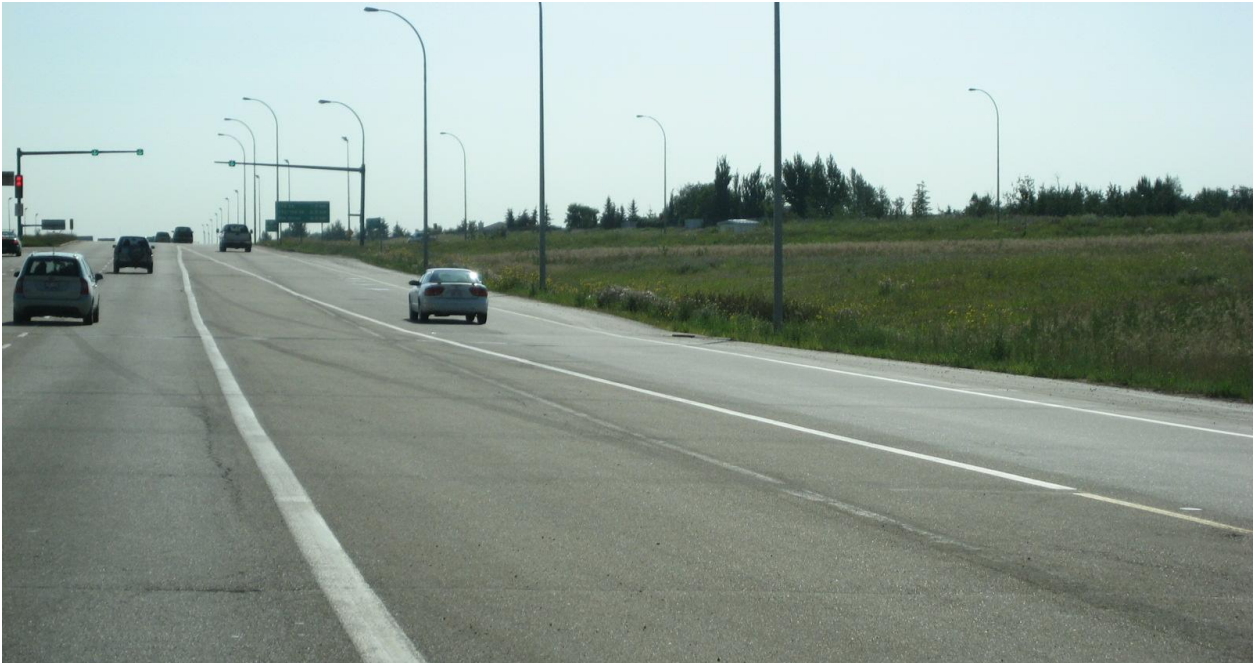
Figure 11: Paved taper requiring hatch-marking
