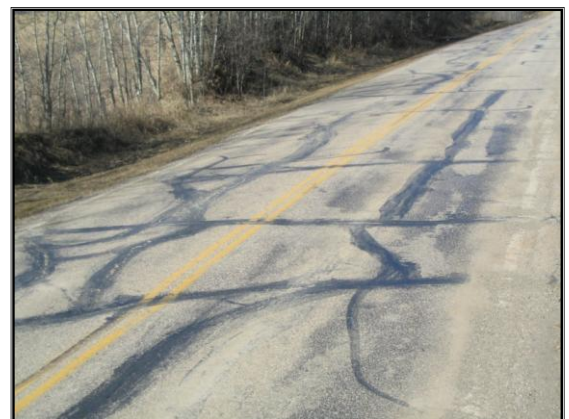
Figure 13 – Block Cracking.
