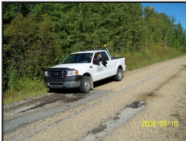
Figure 6 – “In Vehicle” surface rating inspection.
