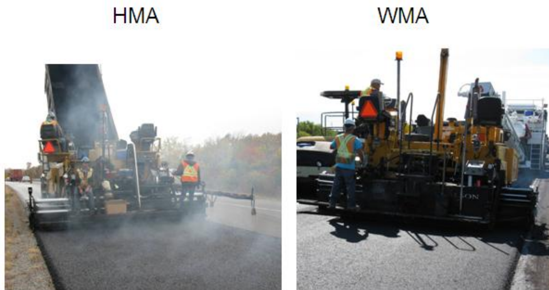
Figure 7: Visible Asphalt Fumes at the Asphalt Paver (HMA vs. WMA)
