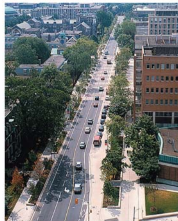
St. George Street running through the heart of the University of Toronto campus was rebalanced in 1997 through the addition of bike lanes and pedestrian-supportive paving treatments to create a street that better supports the many pedestrians and cyclists that use it daily.
