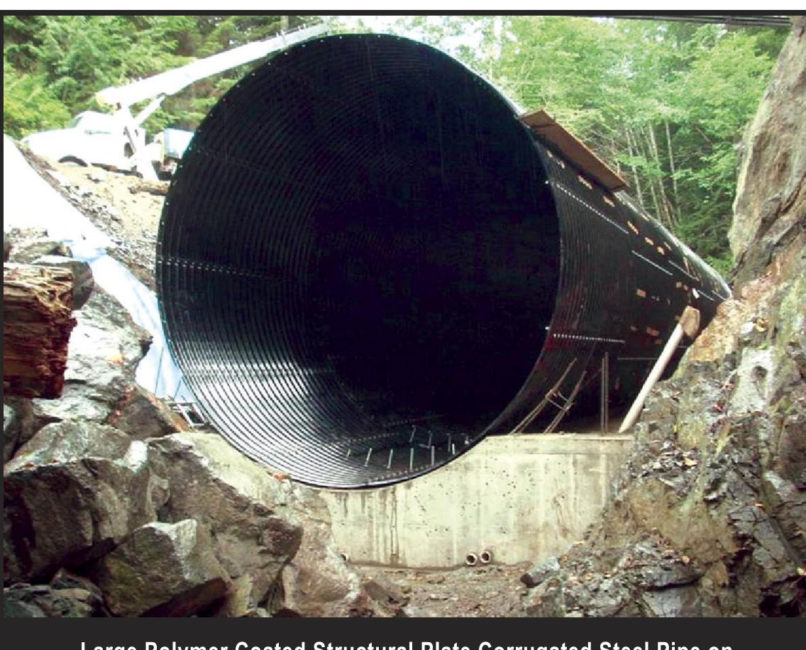
Large Polymer Coated Structural Plate Corrugated Steel Pipe on Vancouver Island in a Severe Level 4 Abrasion Environment Prior to Installation of Sacrificial Concrete Pavement and Fish Baffles
