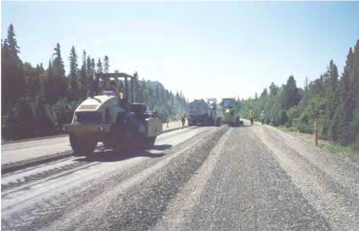
FIGURE 3 The grading and compacting operation following behind the EAS.
