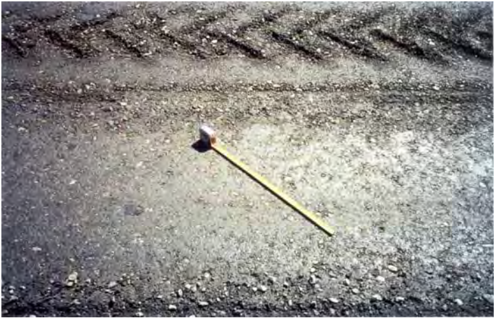
FIGURE 4 The expanded asphalt mat following initial pass of the breakdown roller.
