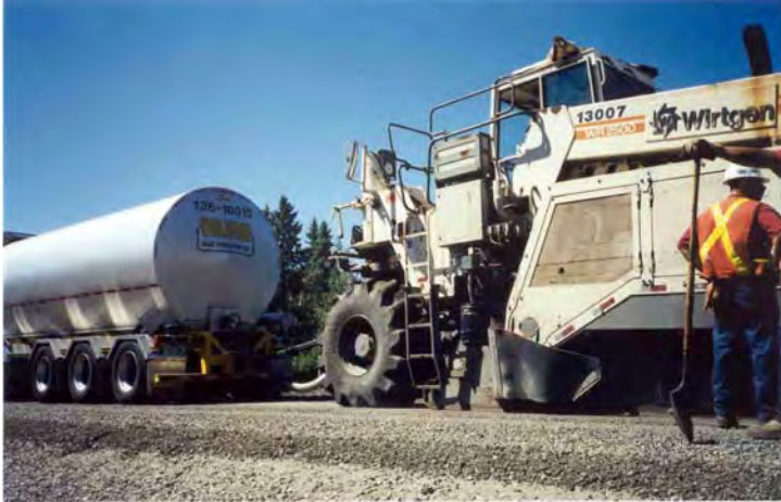
FIGURE 2 The reclaimer/stabilizer attached to a tanker of hot asphalt cement.
