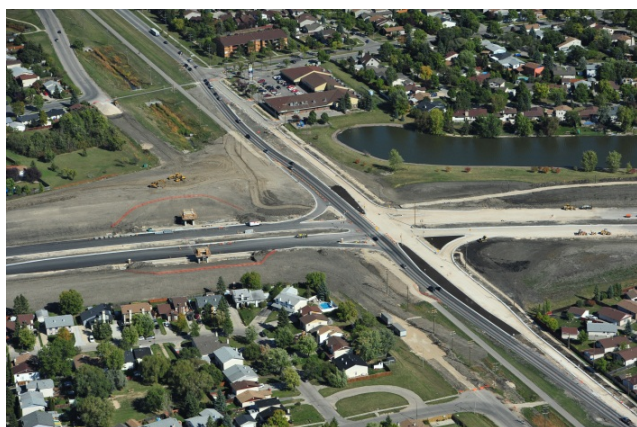
Figure 9: Gateway Road Construction Staging
