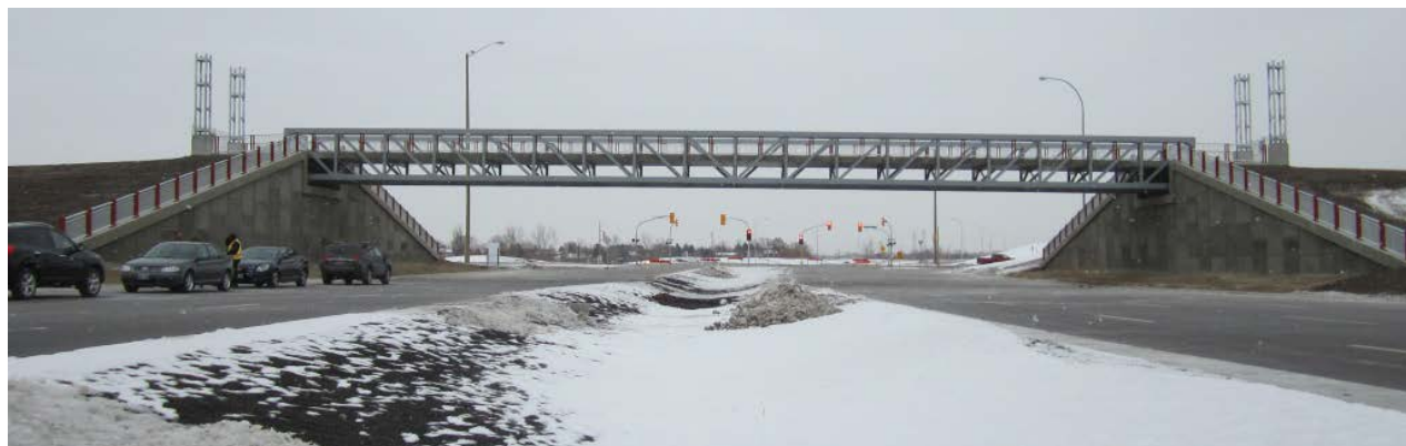
Figure 7: Looking East at Gateway Pedestrian Bridge
