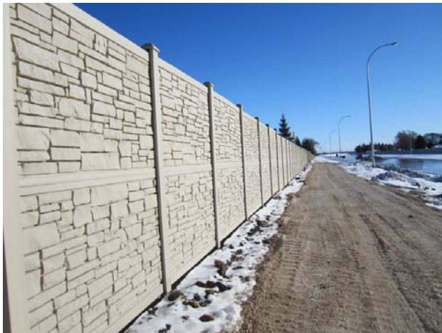
Figure 8: Noise Attenuation Wall
