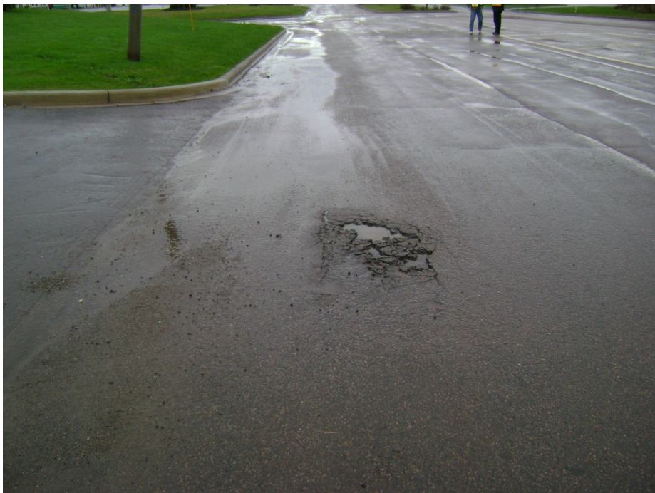
Figure 2: Example of early ravelling.
