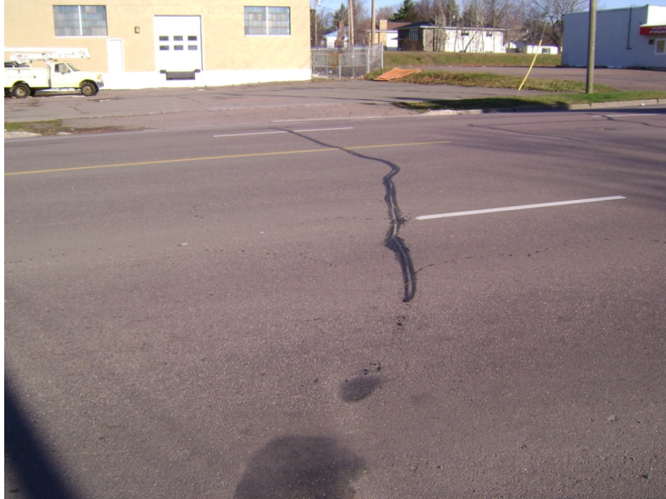
Figure 3: Premature cracking.
