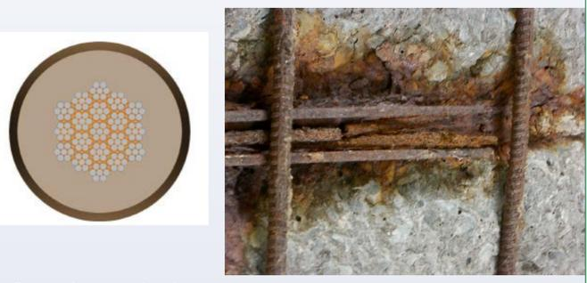
Inner wire corrosion due to the presence of voids and moisture
