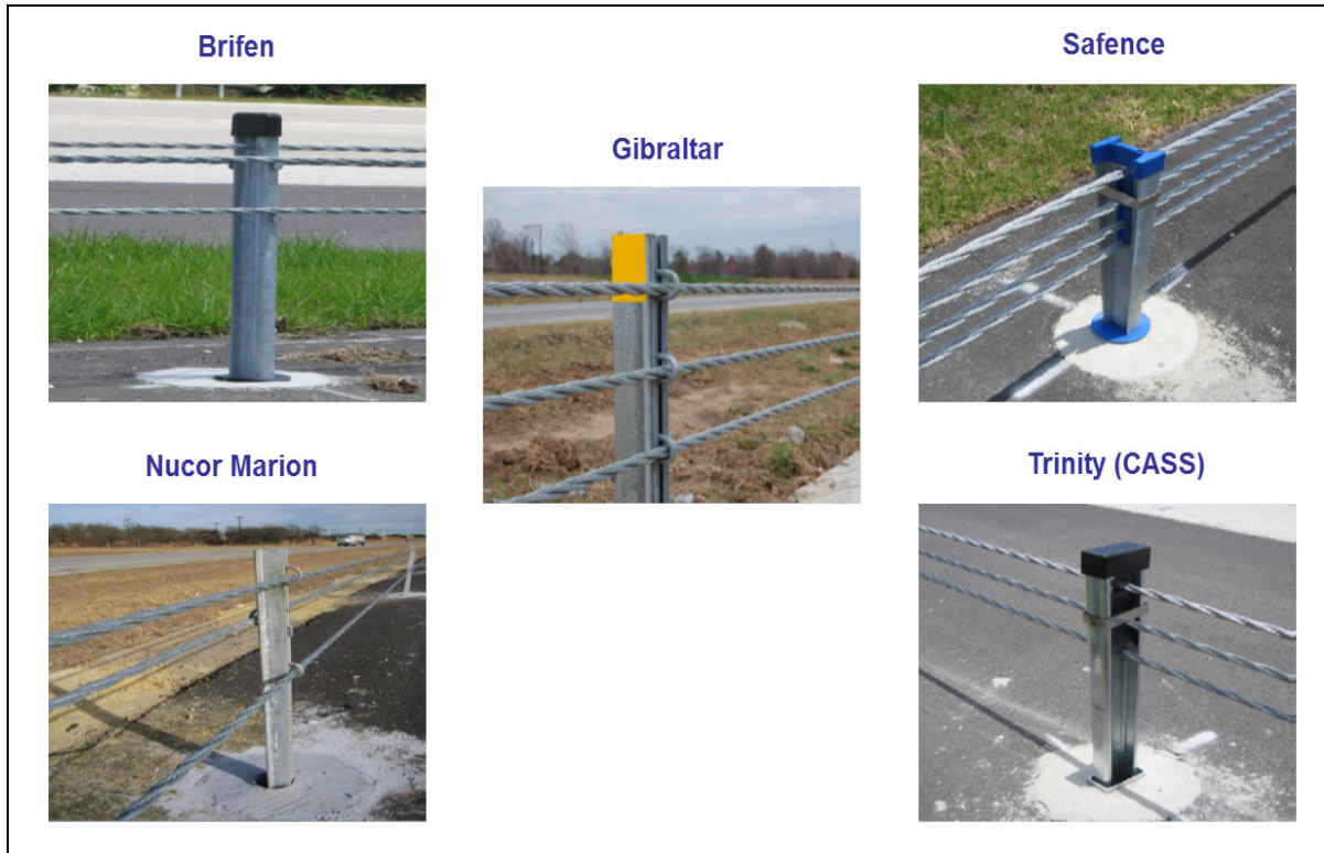
PHOTO 1. Photos of the five FHWA-approved high tension cable barrier systems.
