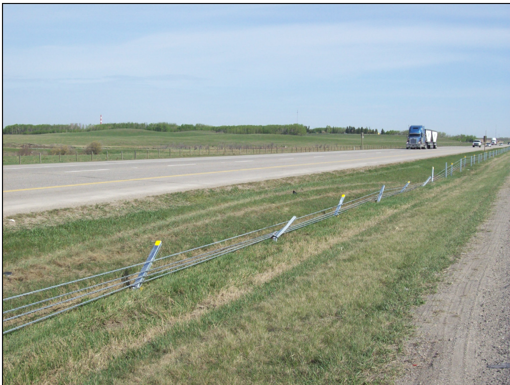
PHOTO 2. Typical HTCB hit in the median of Highway 2 looking downstream (vehicle travelling in direction of photo). Note wheel path in grass.
