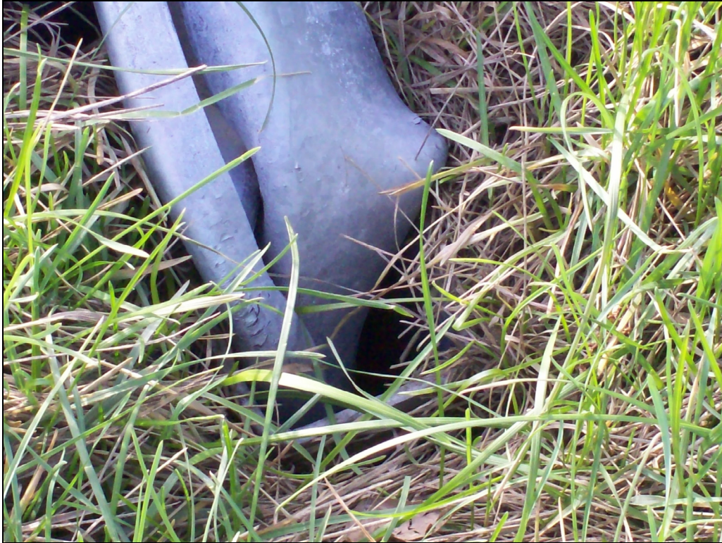
PHOTO 4. Bent post with un-damaged socket can be extracted and a new post fitted.
