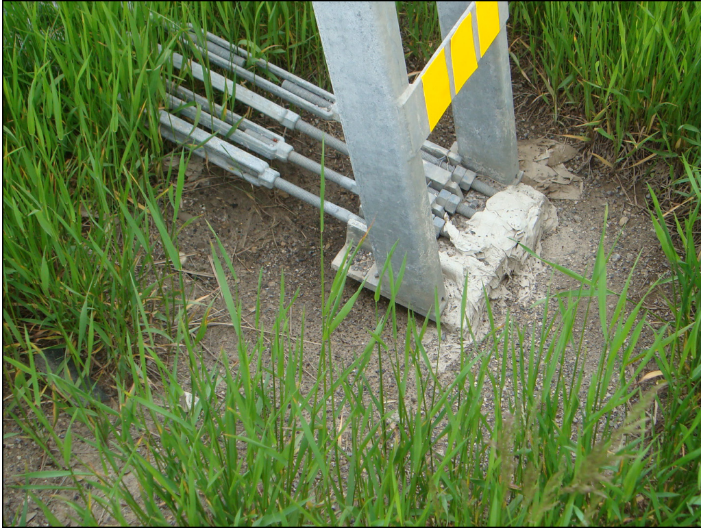
PHOTO 7. Cast in place concrete end terminal anchor with no movement.
