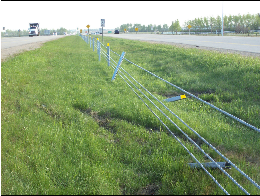
PHOTO 3. Typical HTCB hit in the median of Highway 2 looking upstream (vehicle was traveling toward photo on left side of the median). Note direction of posts.
