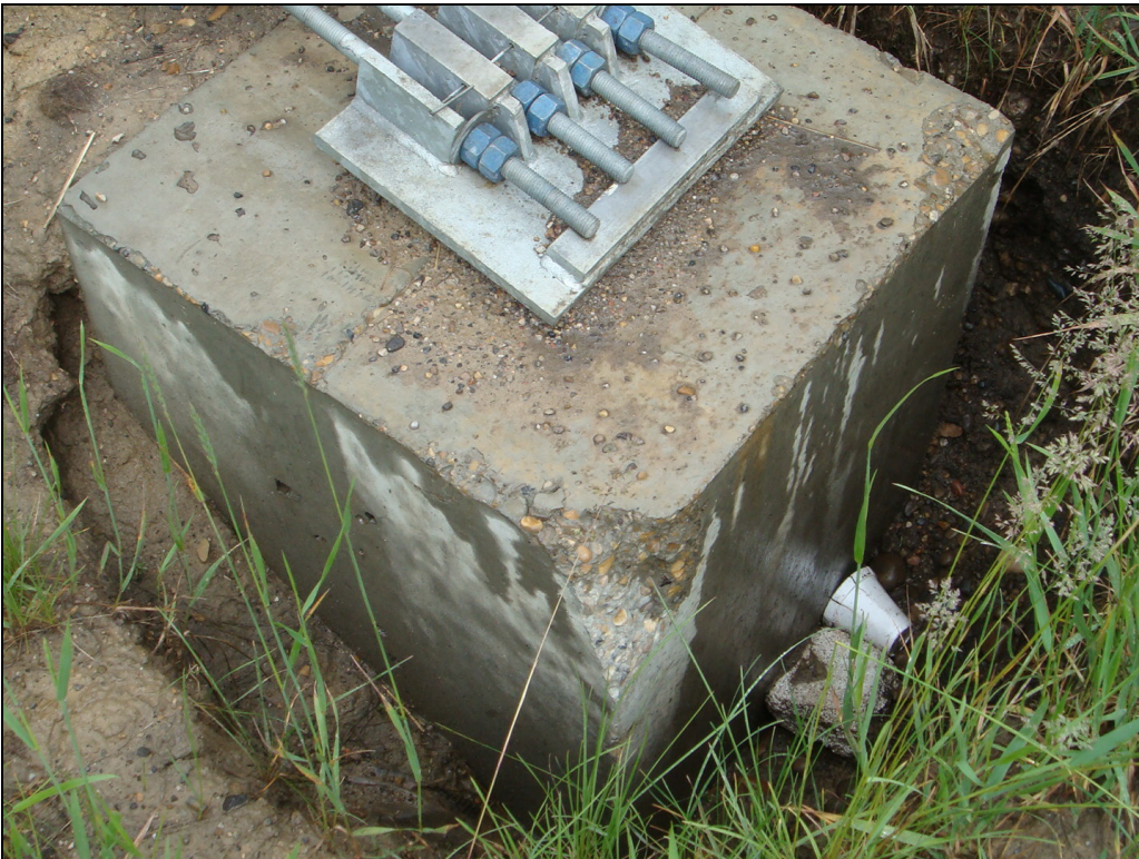
PHOTO 8. Pre-cast concrete end terminal anchor out of plumb and erosion.
