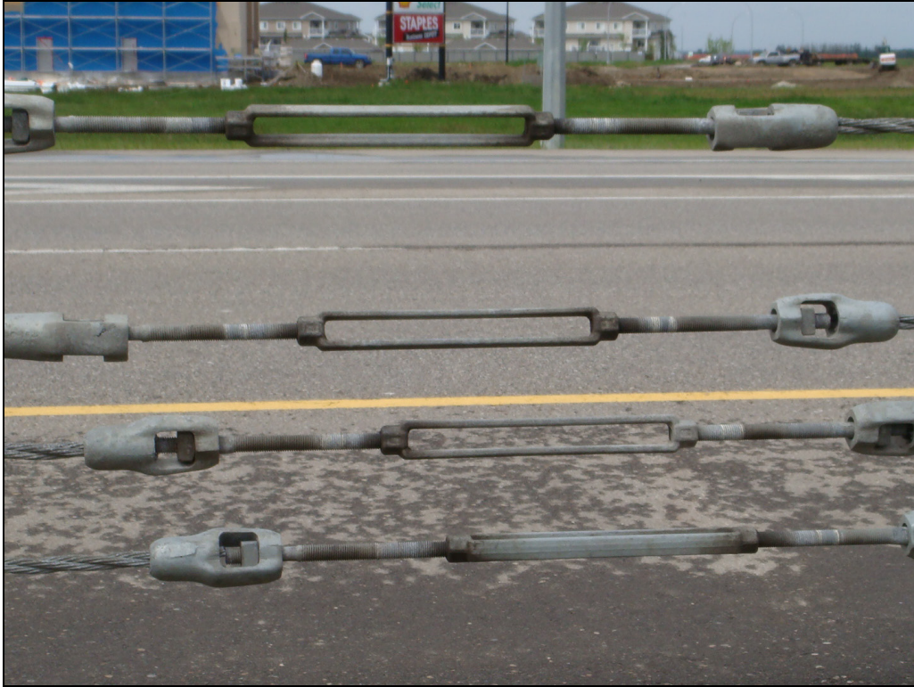
PHOTO 9. Turnbuckles connecting cables with insufficient thread following tension release.
