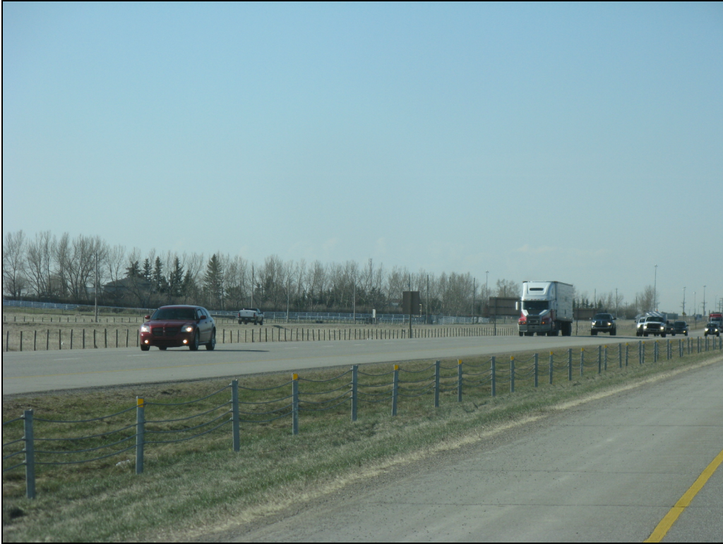
PHOTO 5. Sagging cables due to release of end terminal.
