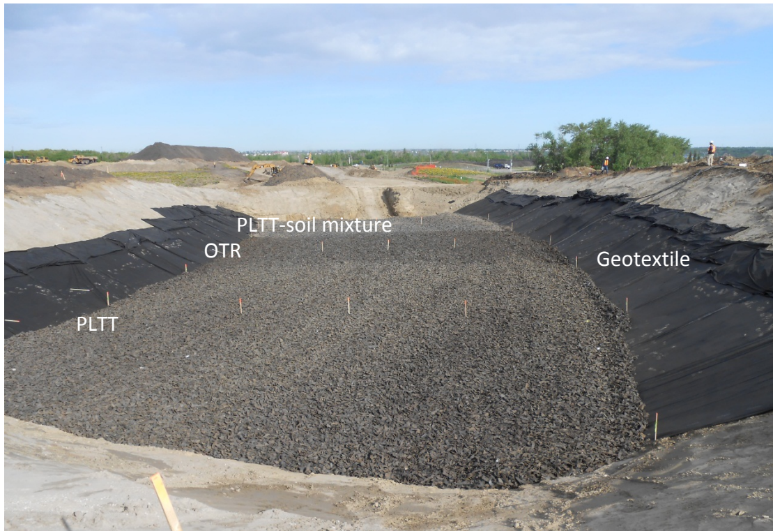
1 2 Figure 4. The embankment pit, half filled with PLTT, OTR and PLTT-soil mixture. 3
