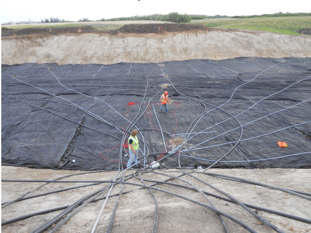
Figure 7. Installation of settlement plates in the three TDA fill embankment test sections.
