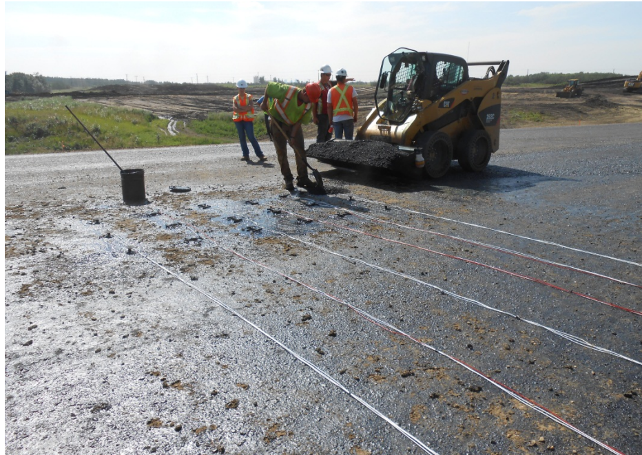
5 6 Figure 9. Asphalt strain gage installation process.
