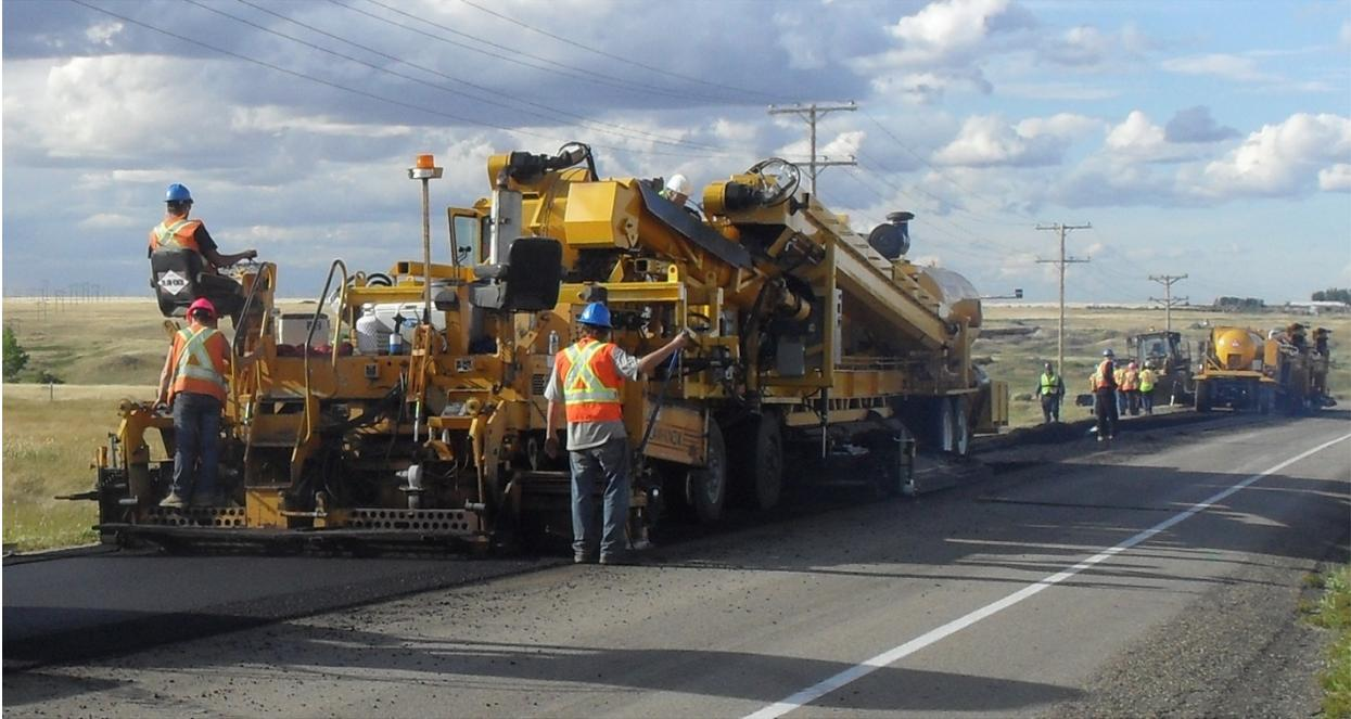
**Picture 1.** HIR surface rehabilitation project in Saskatchewan, Summer 2011 (HIR pug-mill and paver in centre; HIR heater-scarifier unit on far right).
