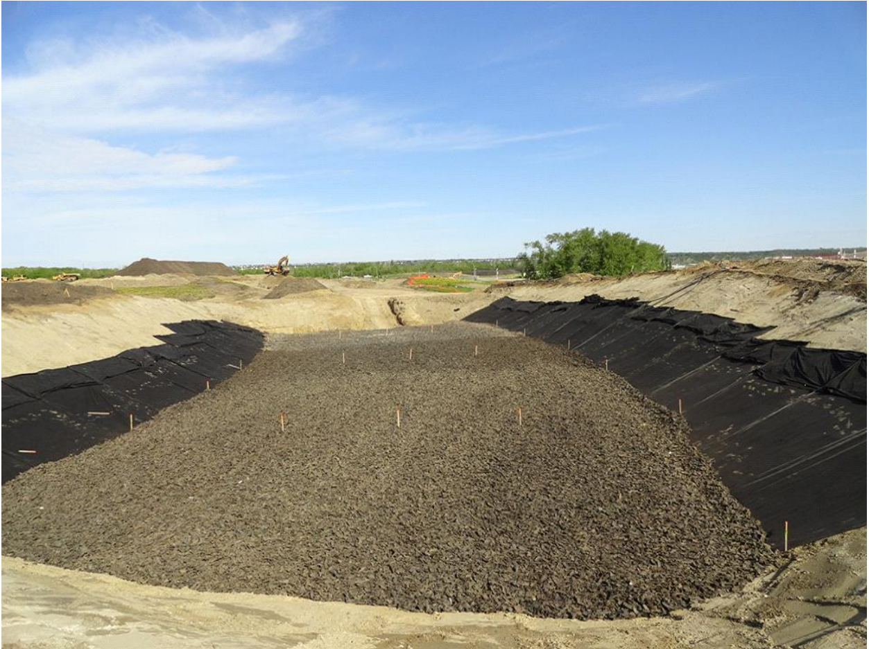
Picture 1. Embankment filled with TDA during construction, summer 2012.
