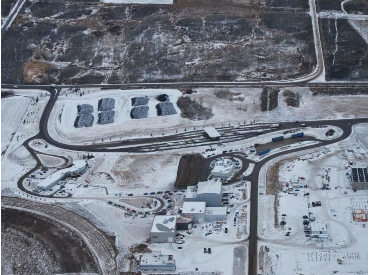
Picture 3 – Stored TDA product for construction project at the Edmonton Waste Management Centre.
