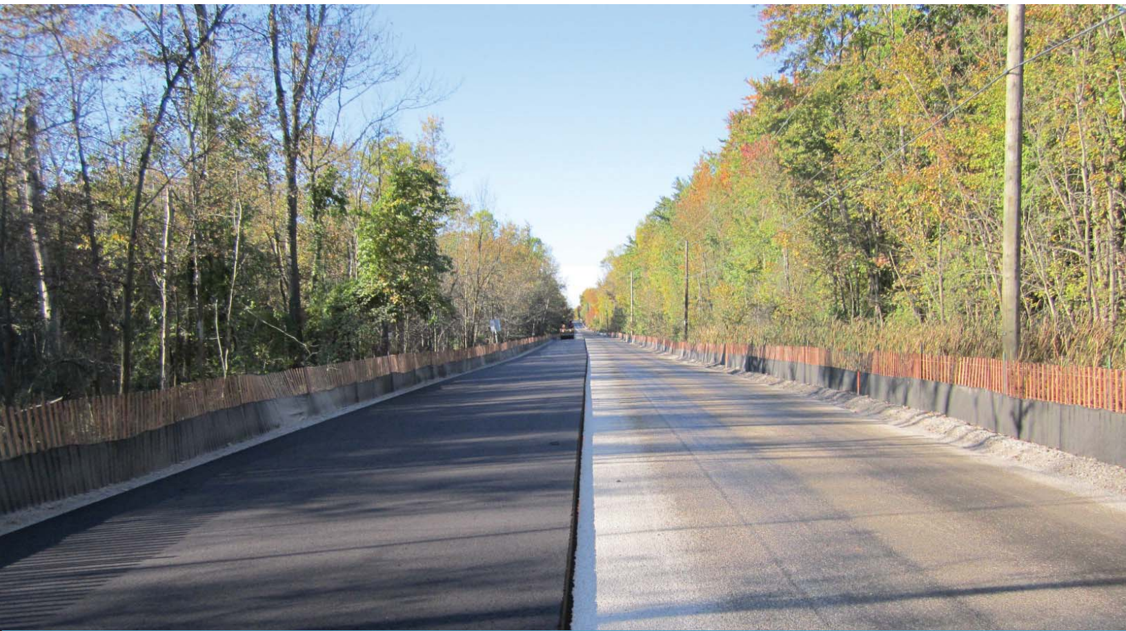
Above: SAMI application and top asphalt on Campbellville Road Below: SAMI application on Steeles Avenue
