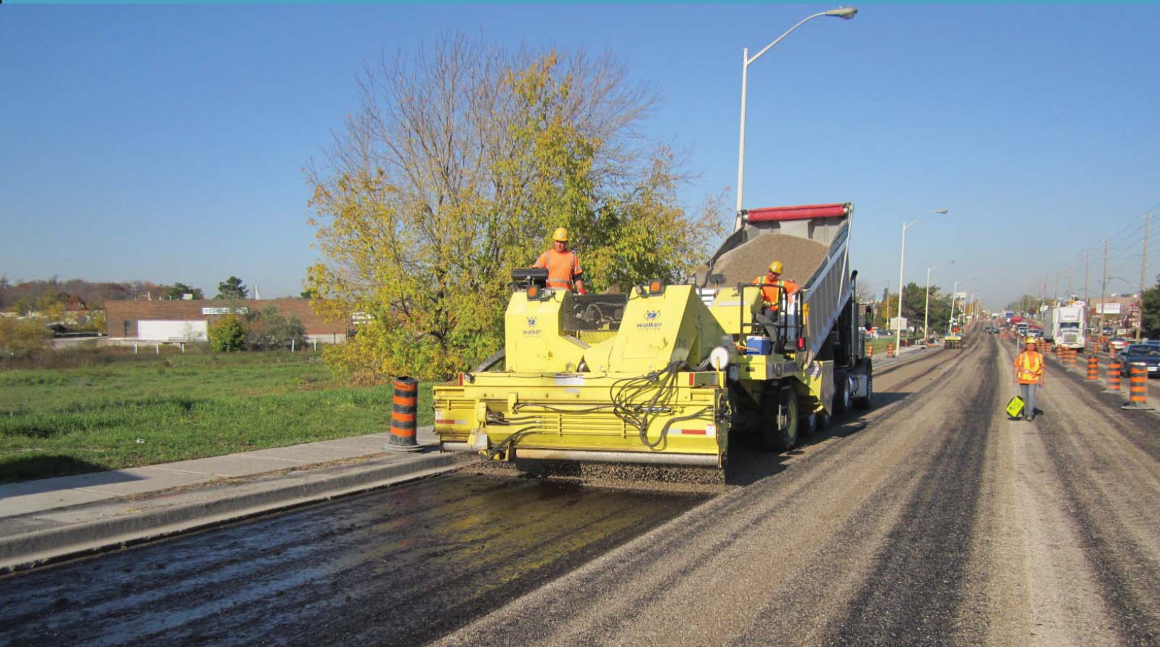
Above: SAMI application and top asphalt on Campbellville Road Below: SAMI application on Steeles Avenue
