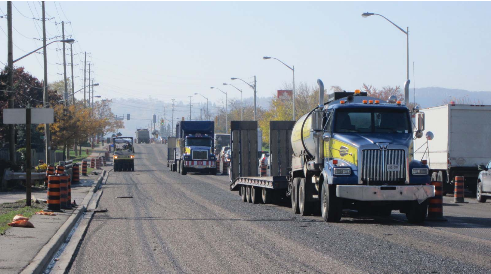
Above: SAMi application on Steeles Avenue Below: Completed resurfacing of Steeles Avenue
