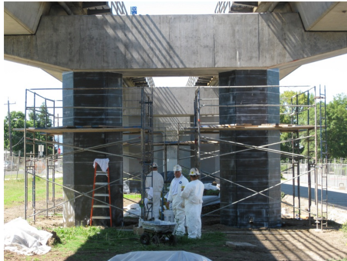
Figure 1: BART C-Line Aerial Structures
