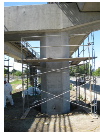
Figure 5: Excavation of Column
