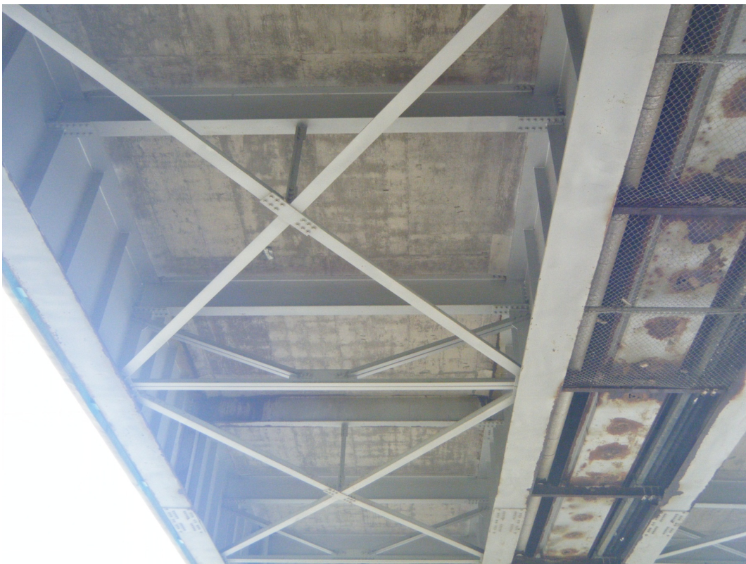
Figure 2 Girders, horizontal cross bracing, floor beams and k-brace diaphragms
