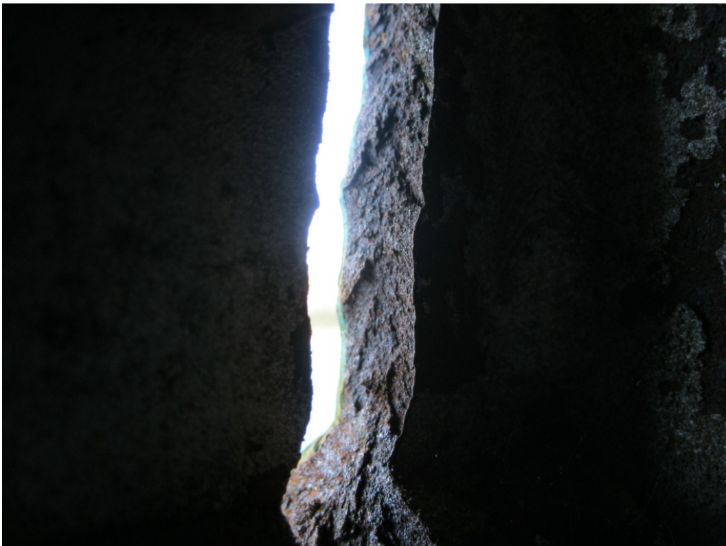
Figure 10 Crack surface and weld fracture
