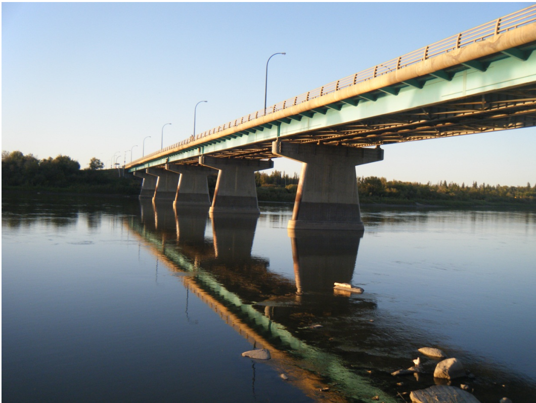
Figure 1 Diefenbaker Bridge, Prince Albert, Saskatchewan
