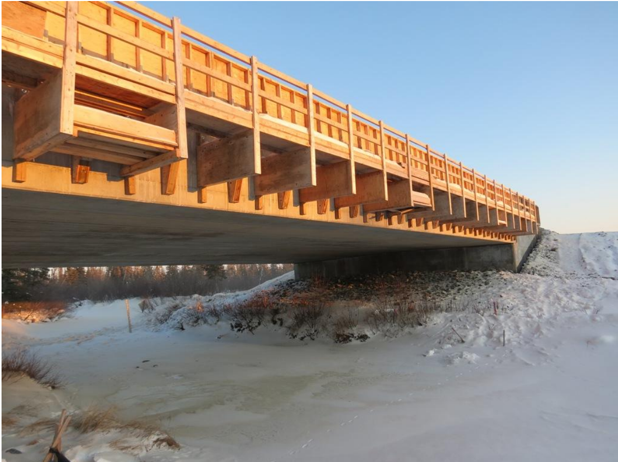
Photo 10: Looking Back Creek Bridge
