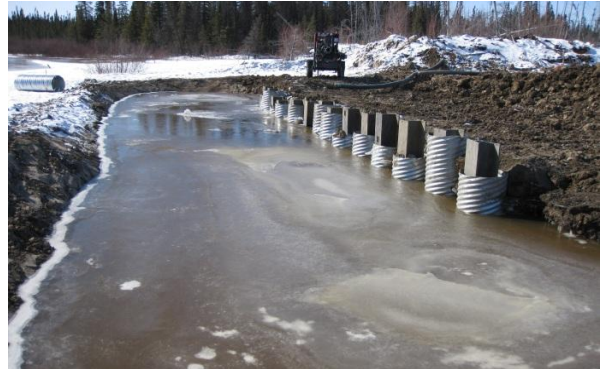
Photo 7: High Water Level During Construction
