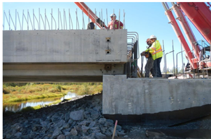
Photo 3: An Upper and Lower Lateral Post-Tensioned Ducts
