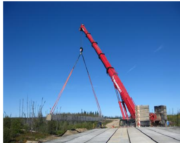
Photo 4: 500 Tons Capacity Mammoet Crane Erecting Girder
