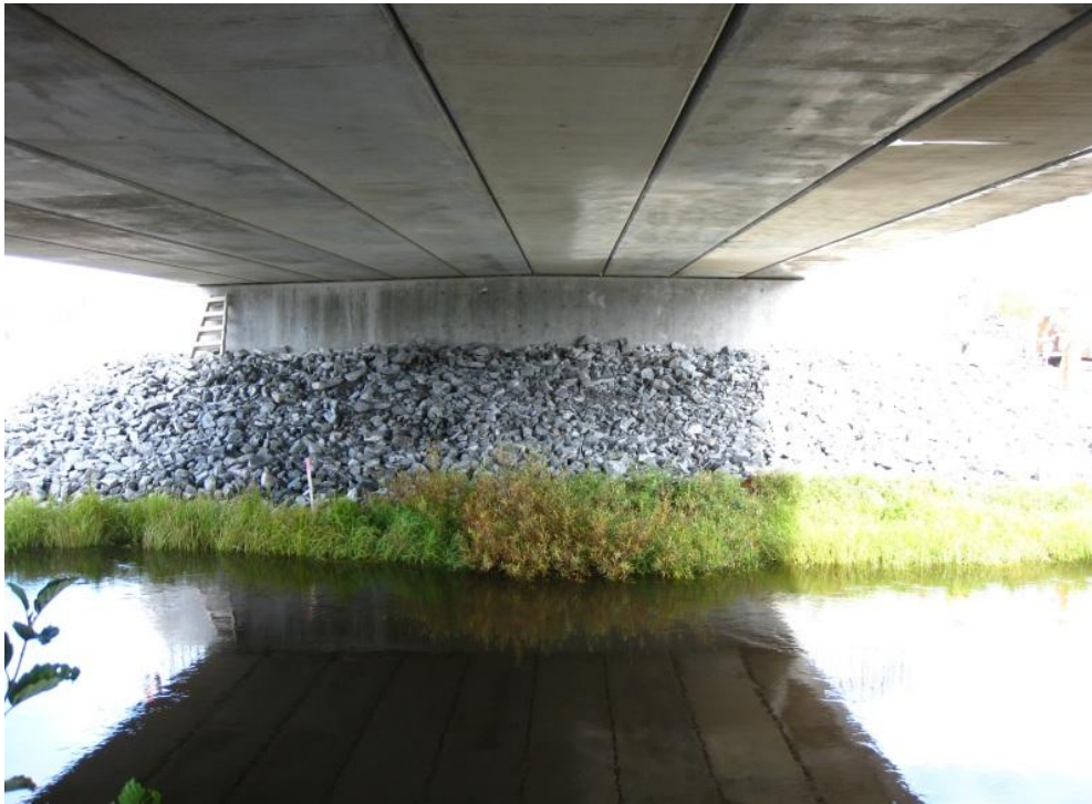
Photo 8: Undisturbed Stream Crossing
