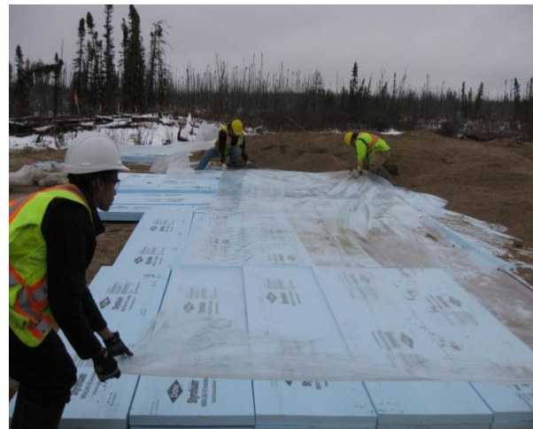
Photo 5: Insulation Installation
