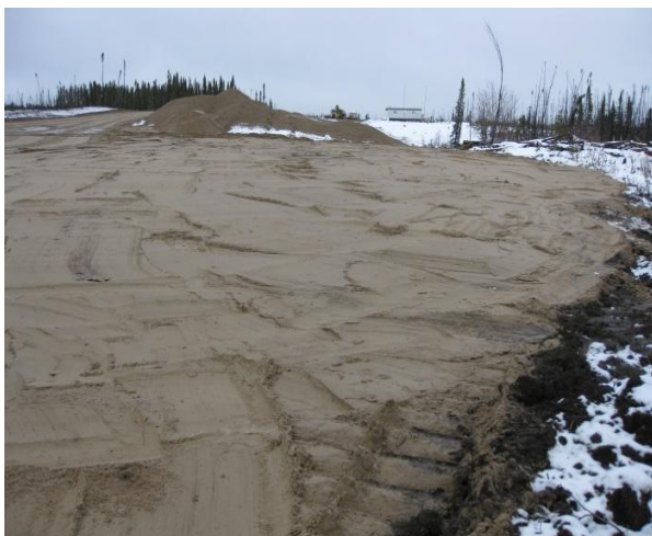
Photo 6: Sand Bedding Installation
