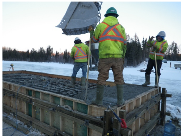
Figure 8: Concrete Placement at Mainland
