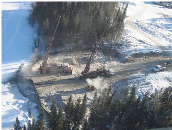
Figure 7: Drill Rigs at Mainland
