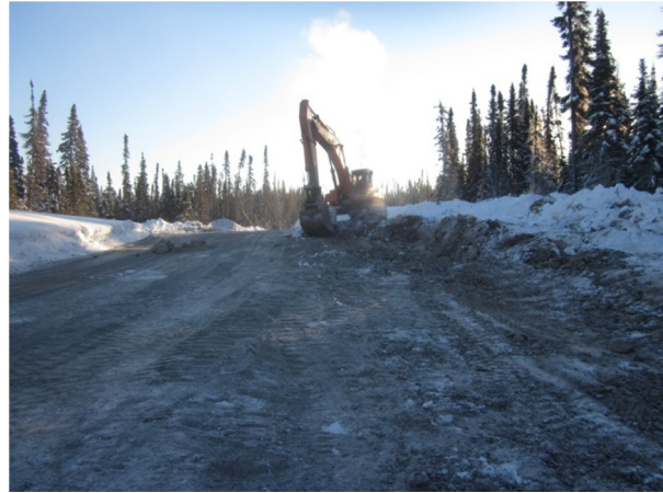
Figure 19: Road Upgrades at Red Sucker
