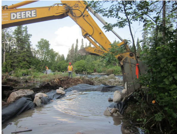
Figure 11: Channel Re-Route at Red Sucker
