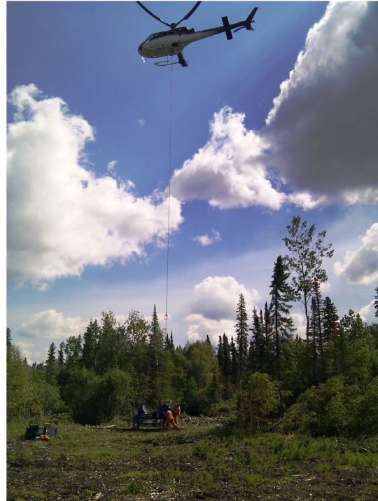
Figure 6: Drill Rig Assembly at Red Sucker
