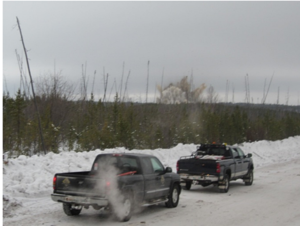
Figure 20: Blasting at the Quarry at Feather Rapids
