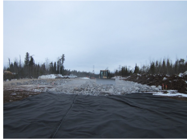
Figure 21: Sewn Geosynthetic at Feather Rapids
