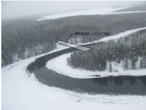
Figure 2: Mainland River Bridge Location
