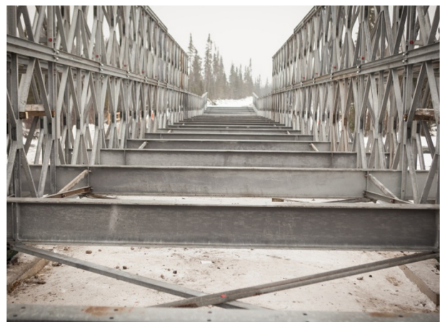
Figure 14: Acrow Construction at Red Sucker
