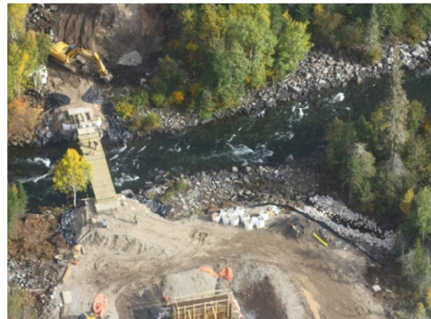
Figure 12: Channel Re-Route at Red Sucker
