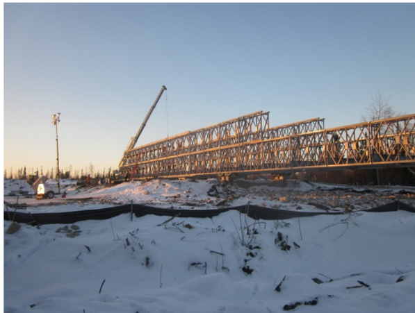
Figure 13: Acrow Construction at Red Sucker
