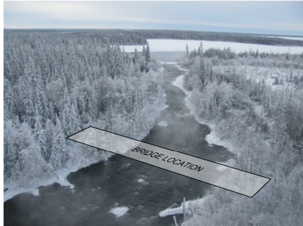
Figure 3: Red Sucker River Bridge Location
