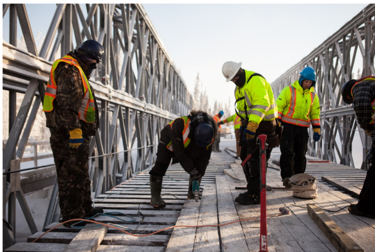
Figure 7: Timber Deck Assembly at Red Sucker
