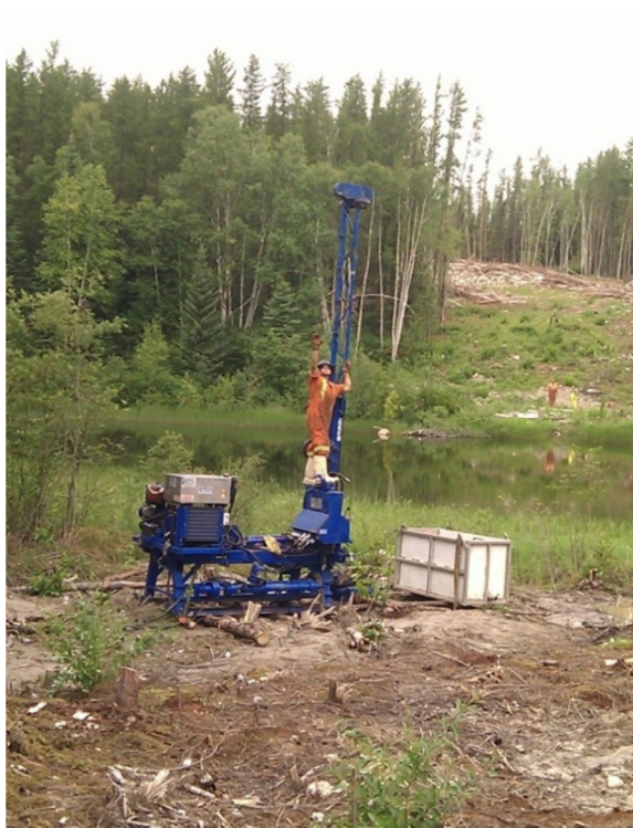
Figure 5: Drill Rig Assembly at Mainland River
