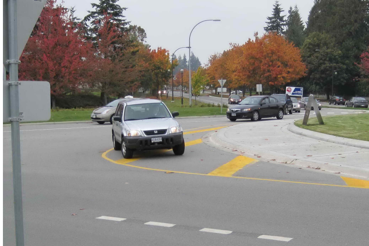
Figure 3.3 Example of Ineffective Circulatory Road Markings. Drivers can run over the markings and end up in the incorrect circulating lane.
