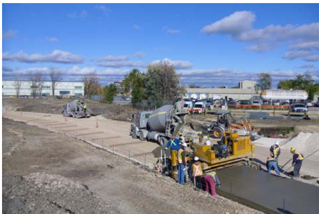
Figure 15 – Slip Form Paving of Transit Corridor
