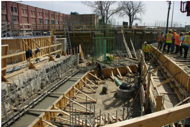
Figure 11 – Construction of Foundations for Bridge Substructure
