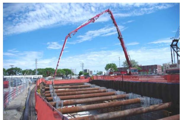
Figure 9 – Installation of Shoring System
