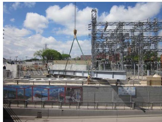
Figure 12 – Erecting Bridge Girders for Superstructure
