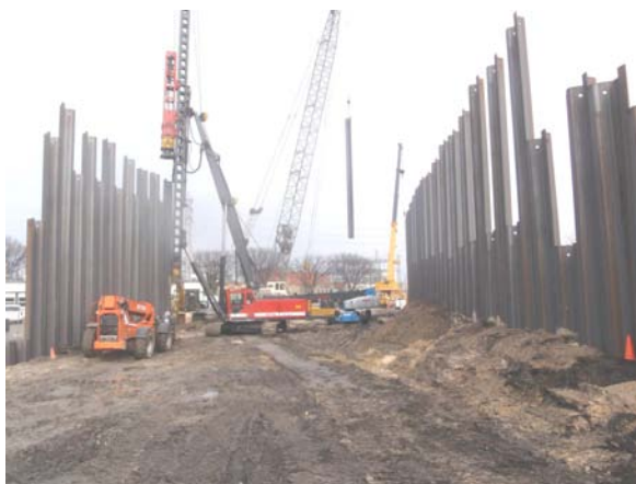
Figure 8 – Tunnel Sheet Piling Installation
