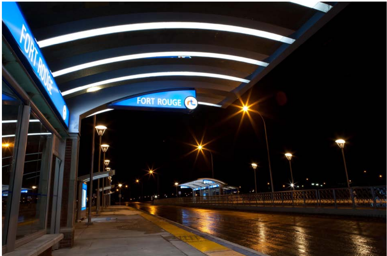
Figure 17 – Completed Fort Rouge Station
