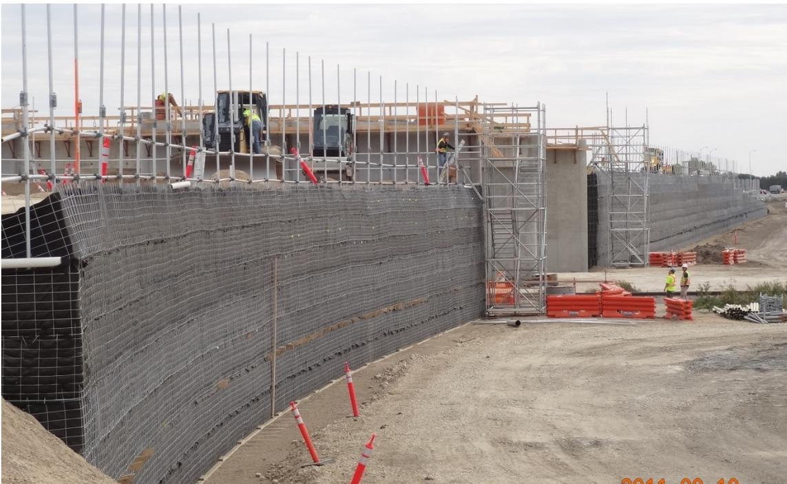
*Figure 3 – MSE Wall Construction*
