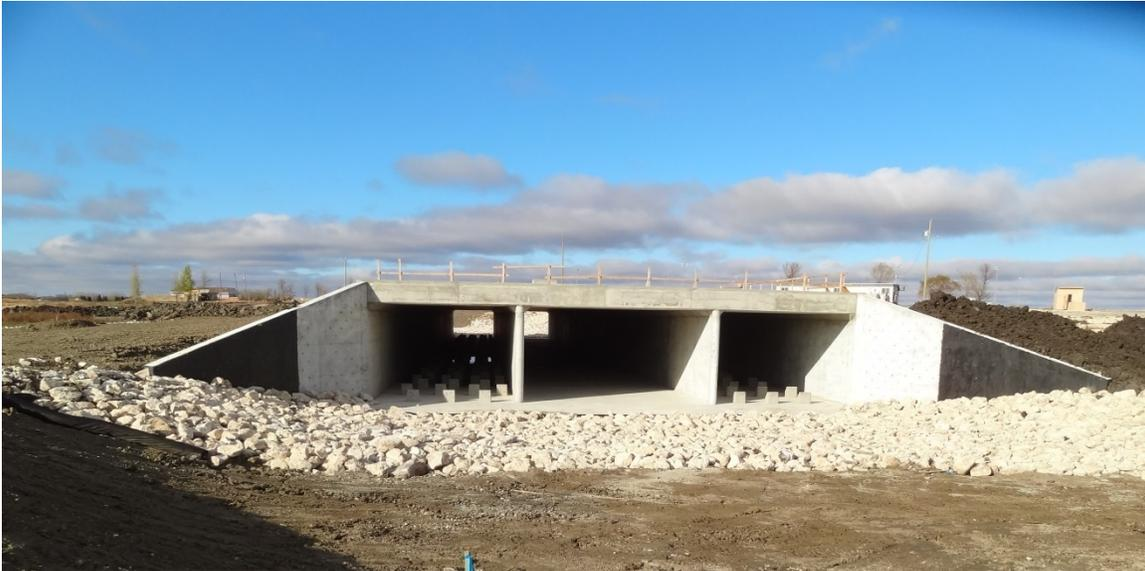
*Figure 10 -Structure 3 with Cast-in-Place Rip Rap in Exterior Cells for Fish Passage*
