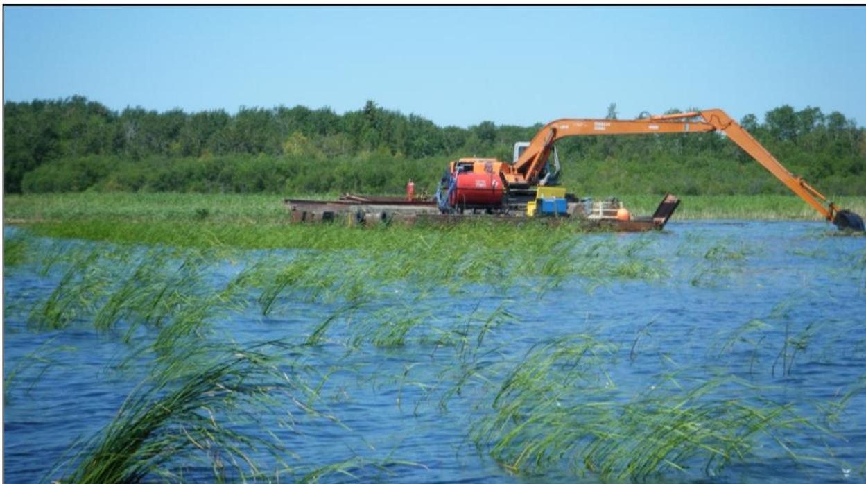
Figure 6 – Access Channel Construction Using Barge Mounted Excavator
