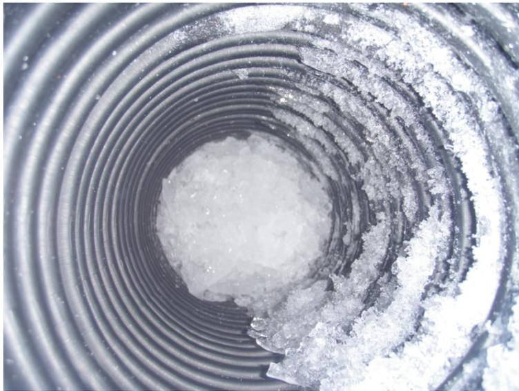
Figure 14: Ice chunks accumulation were observed in most ventilation chimneys
