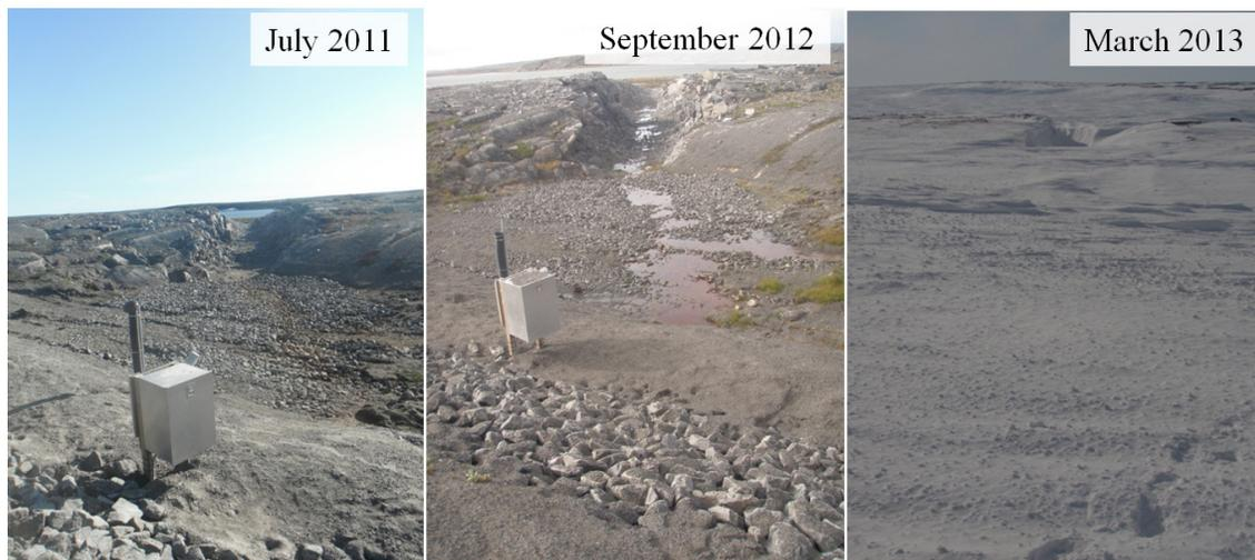
Figure 12: Convective embankment on the east side at different time, with view towards the water deviation channel
