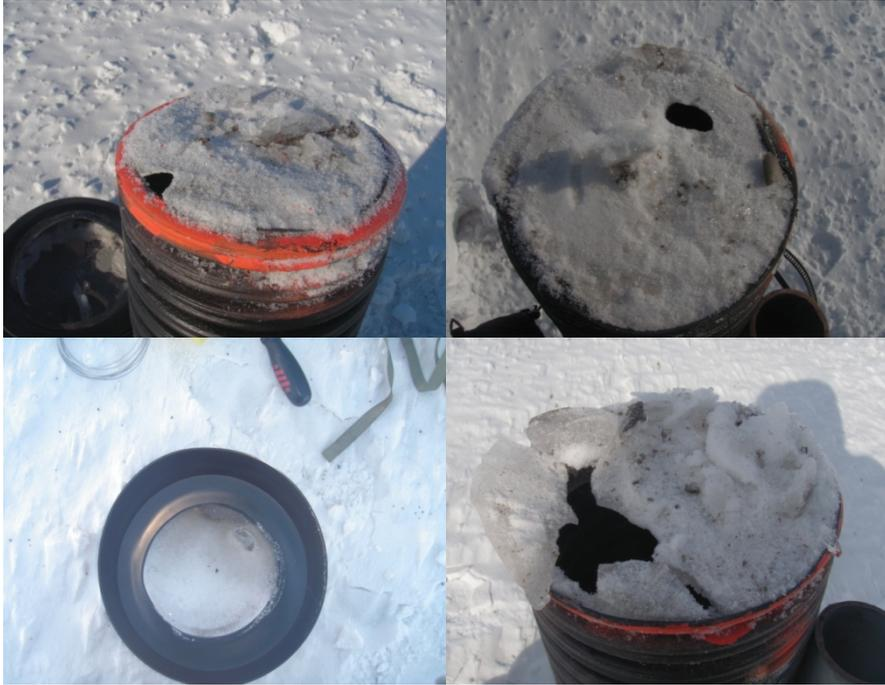
Figure 13: Ice covers forming under the ventilation covers
