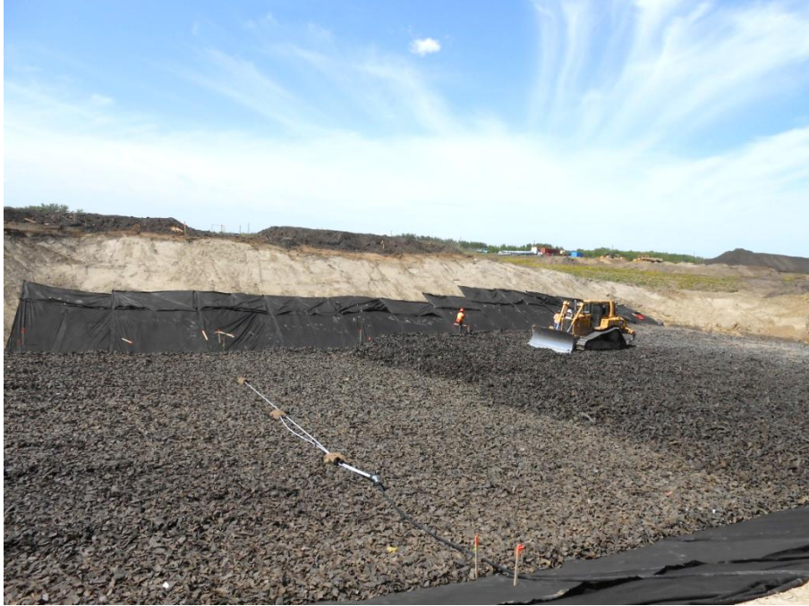
Figure 3 Picture of the test embankment during construction and instrumentation.
