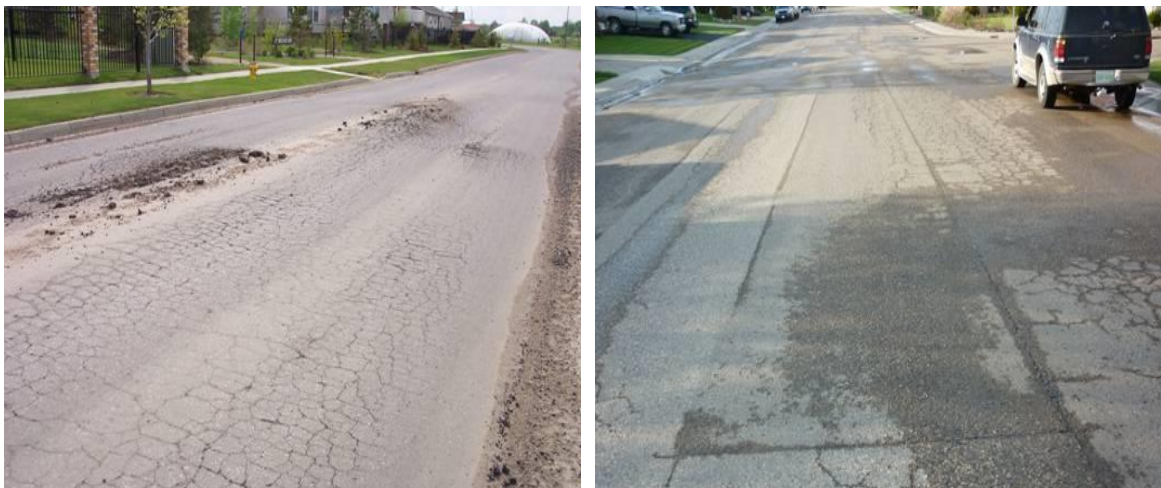
a) Failure of a 7-Year-Old Road
