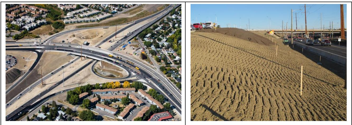
Photo 14 (L) Aerial view of interchange requiring ESC controls; Photo 15 (R) ground view of ESC controls
