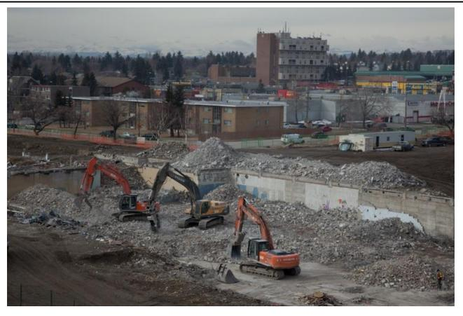
Photo 8 (L) Construction material waste stream separation; Photo 9 (R) Demolition waste stream separation
