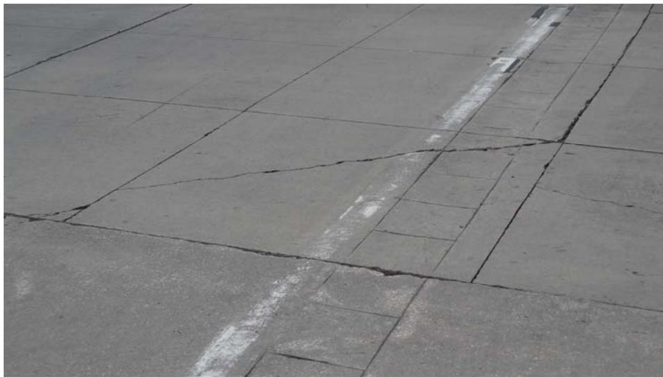
**FIGURE 9 Cracked slabs in crosswalk area.**
