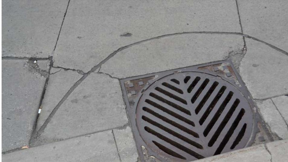
**FIGURE 8 Cracking near catchbasin.**
