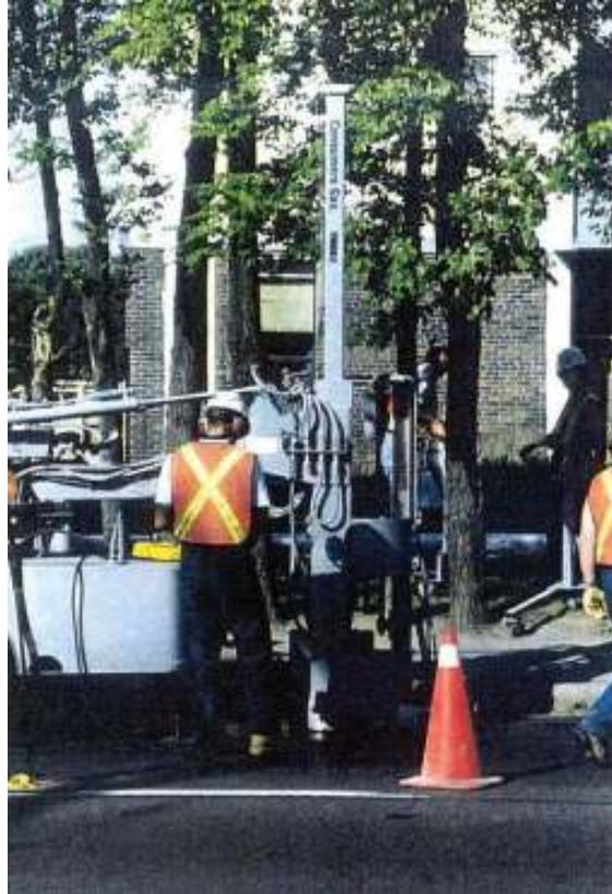
Figure 8 - View of coring rig at 720 Kennedy Road in 1995
