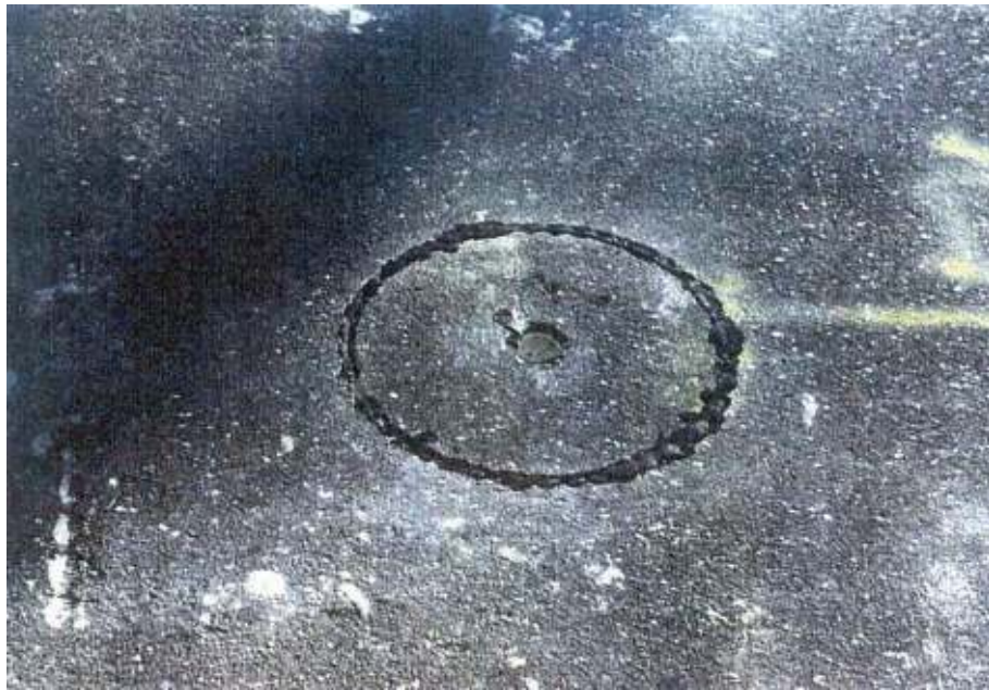
Figure 11 – Close-up view of reinstatement two weeks after installation
