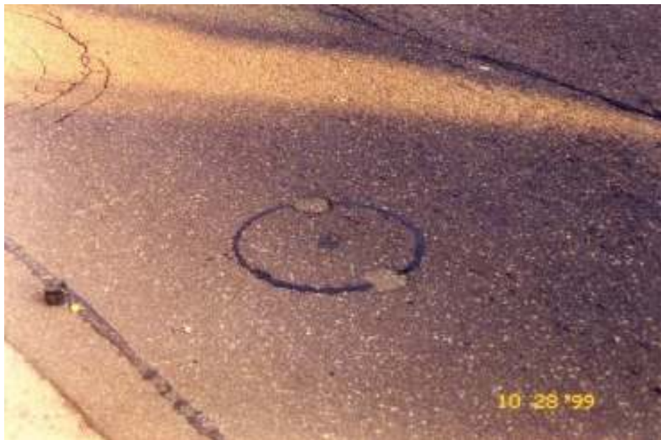
Figure 14 – Close-up view of core on Kennedy Road four years after reinstatement
