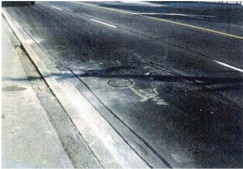
Figure 10 – View of reinstatement two weeks after installation
