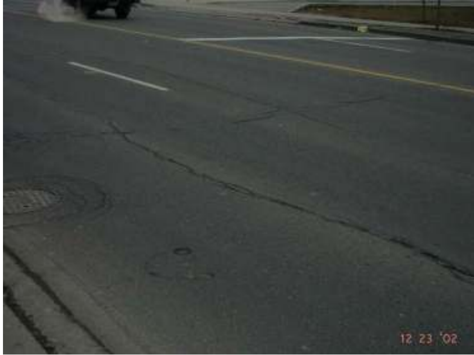
Figure 15 – Kennedy Road Keyhole Core, over seven years after reinstatement (Dec. 2002)
