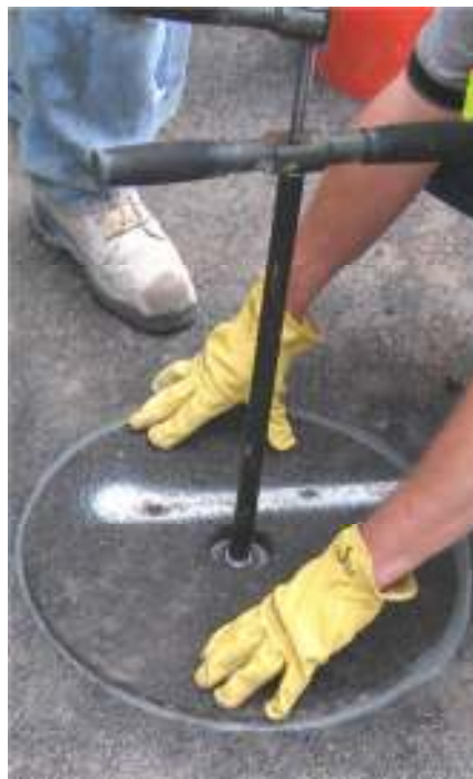
Figure 7 – Final seating of the keyhole core into the pavement
