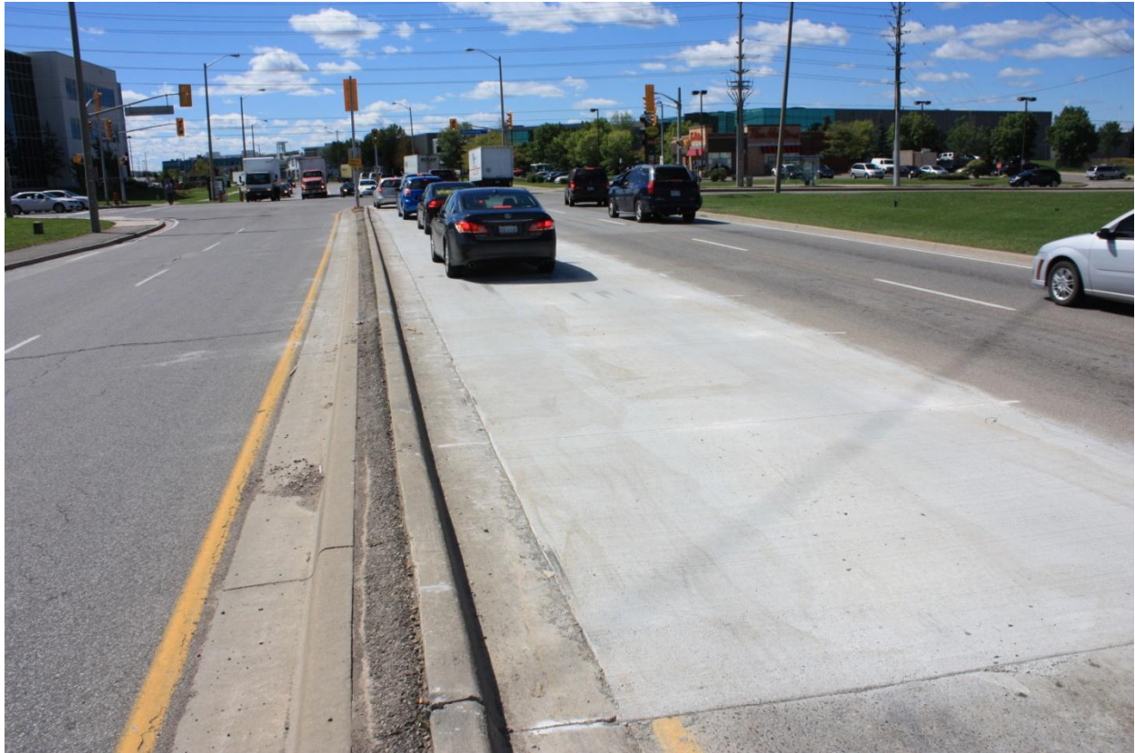
Picture 3: Completed Project September 2012. Source: RMCAO
