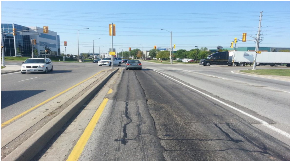
Picture 2: Intersection in August 2012 prior to repair. Source: RMCAO
