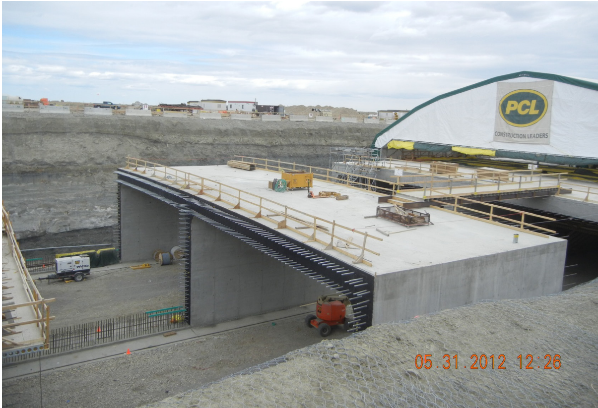
FIGURE 9 – CONSTRUCTED MOVEMENT JOINT
