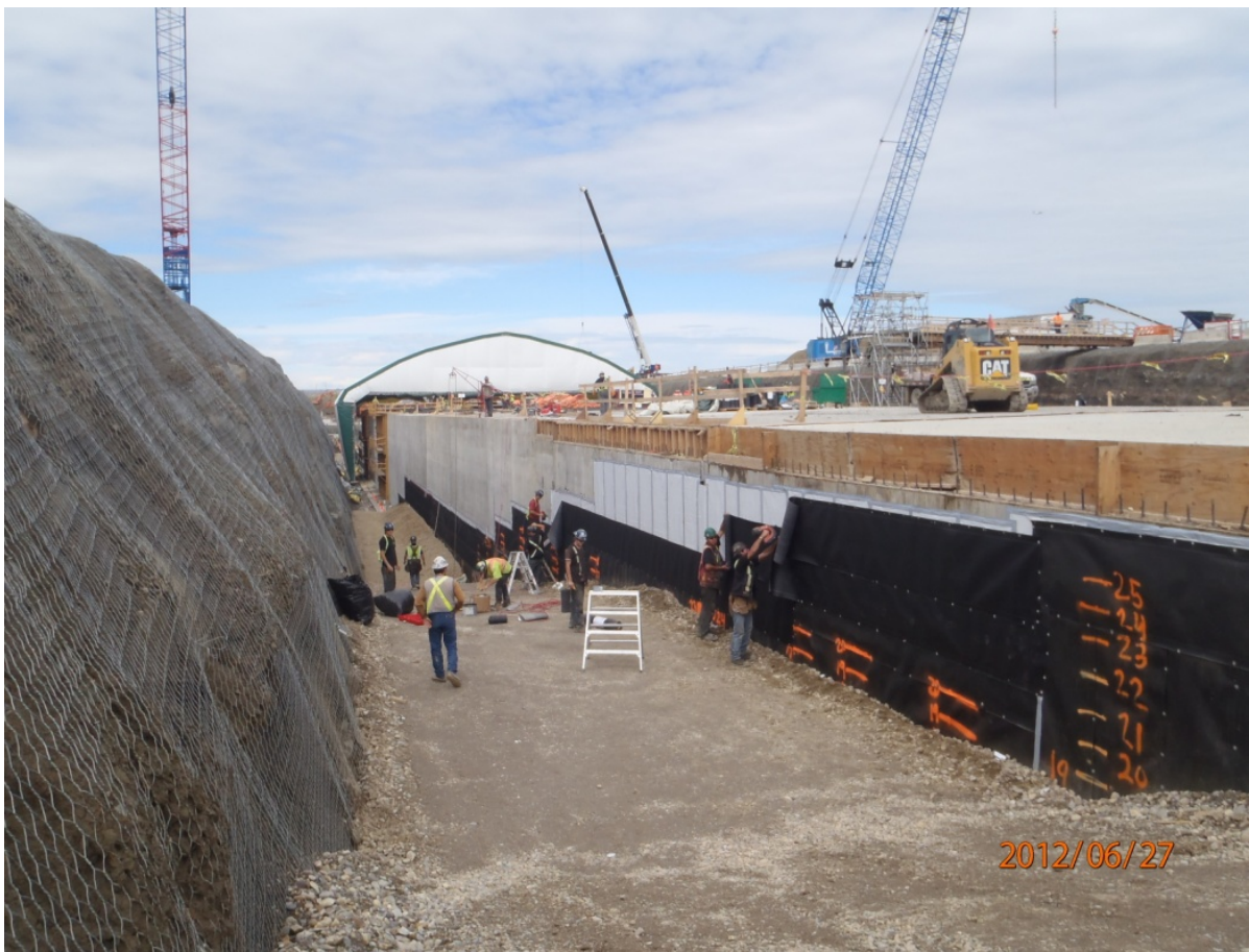
FIGURE 10 – TUNNEL WATERPROOFING SYSTEM
