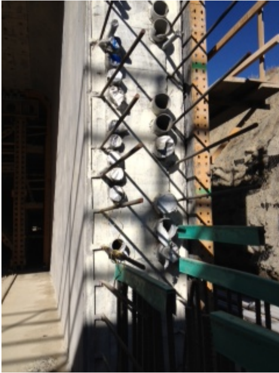
FIGURE 11 – CONDUITS IN TUNNEL WALLS
