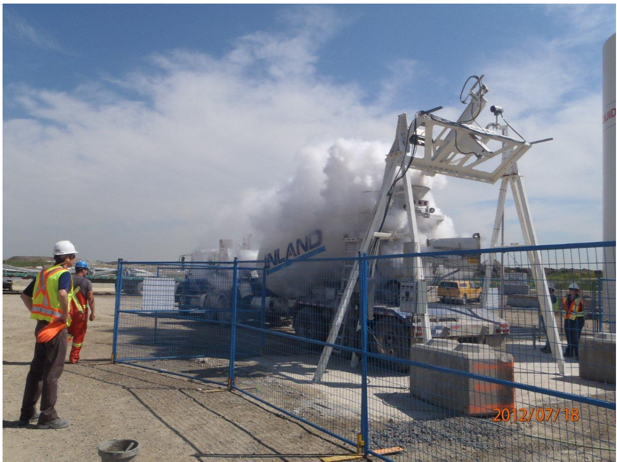
FIGURE 12 – LIQUID NITROGEN INJECTION
