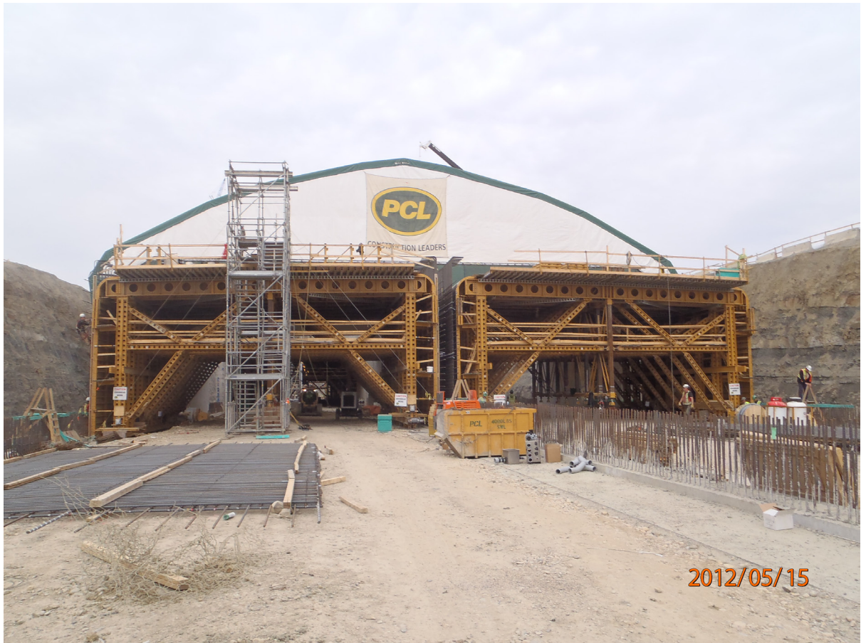
FIGURE 6 - METAL FORMS AND HORDING TENT USED FOR TUNNEL CONSTRUCTION
