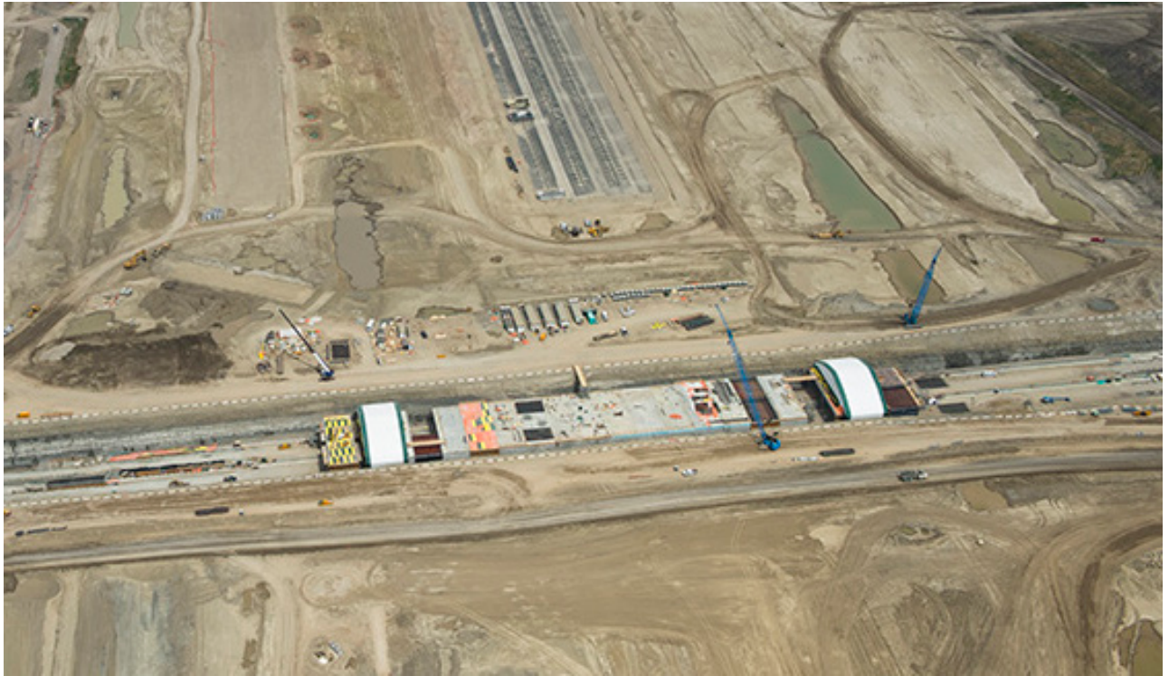
FIGURE 7 – TUNNEL DURING CONSTRUCTION, MAY 2012, LOOKING NORTH
